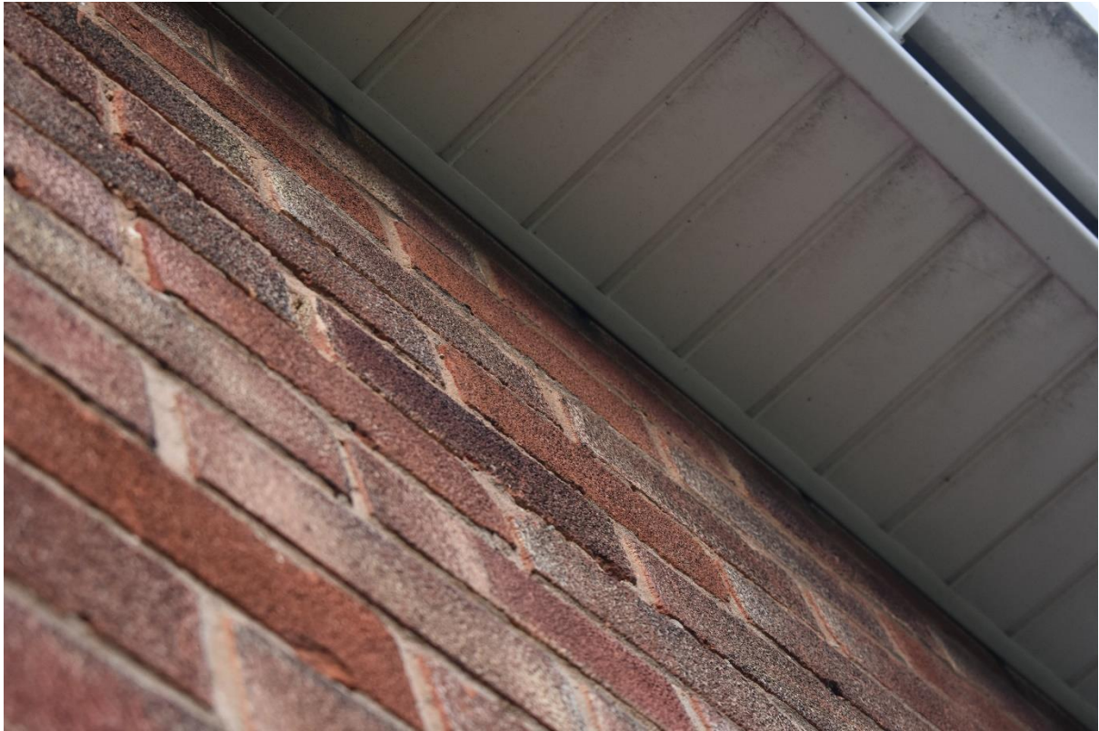
Figure 3.5: The tightly fitted soffits of the dwelling.
