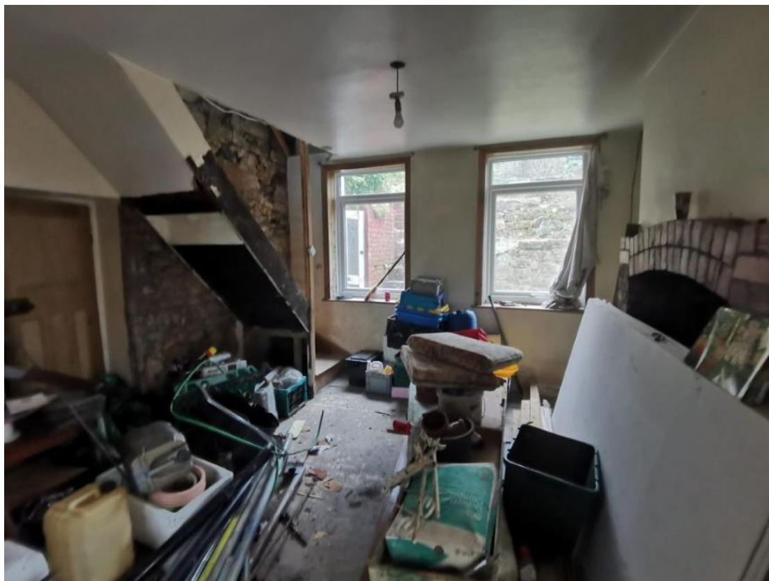
Plate 9 – The ground floor living space of B1.
