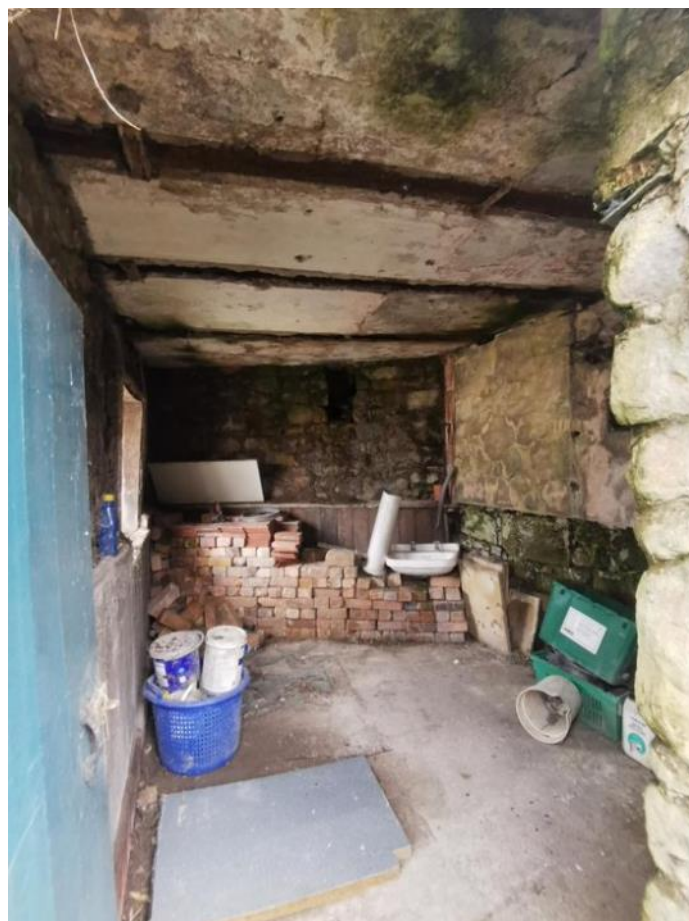
Plate 12 – Internal view of B2 evidencing storage of building materials.
