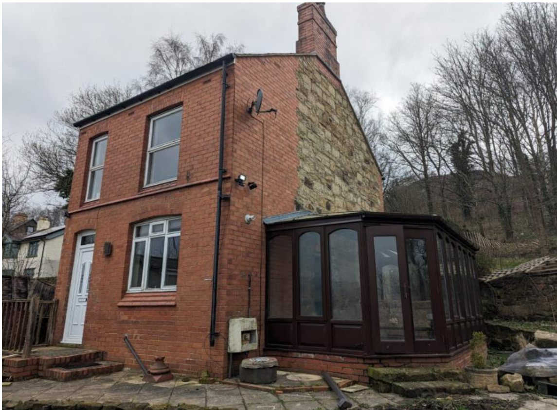
Plate 1 – South-western elevation of B1 at Oakdale.
