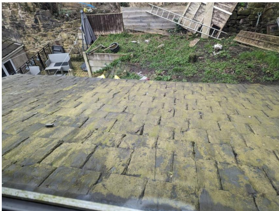
Plate 5 – The roof of the single-storey extension on the northern aspect of B1.
