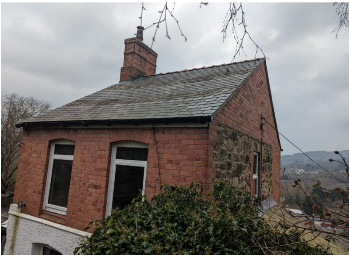
Plate 2 – North-eastern elevation of B1 at Oakdale
