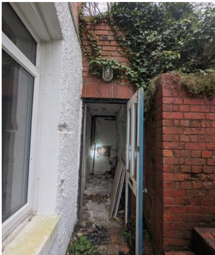
Plate 3 – The attached single-storey outhouse.
