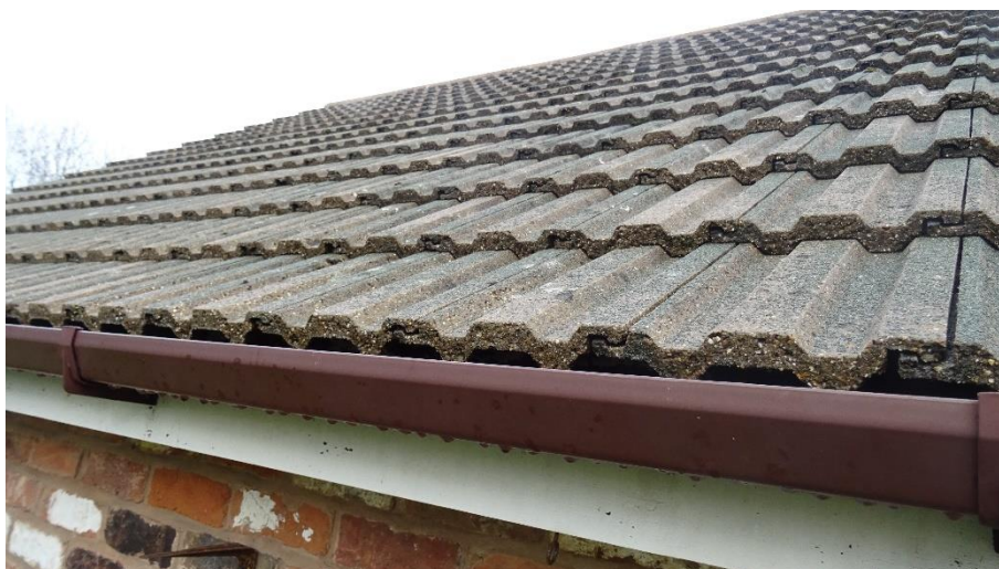
Figure 4.7. Well-set tiles with no potential access points
