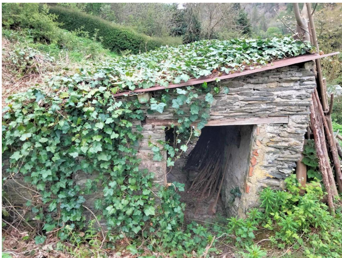
Rear garden: existing out-building to be retained for habitat value
