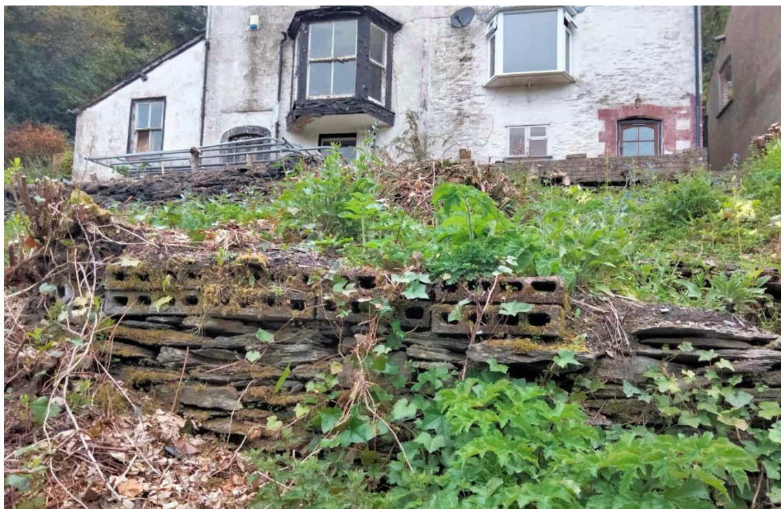
Rear garden: existing drystone wall features to be retained for habitat value
