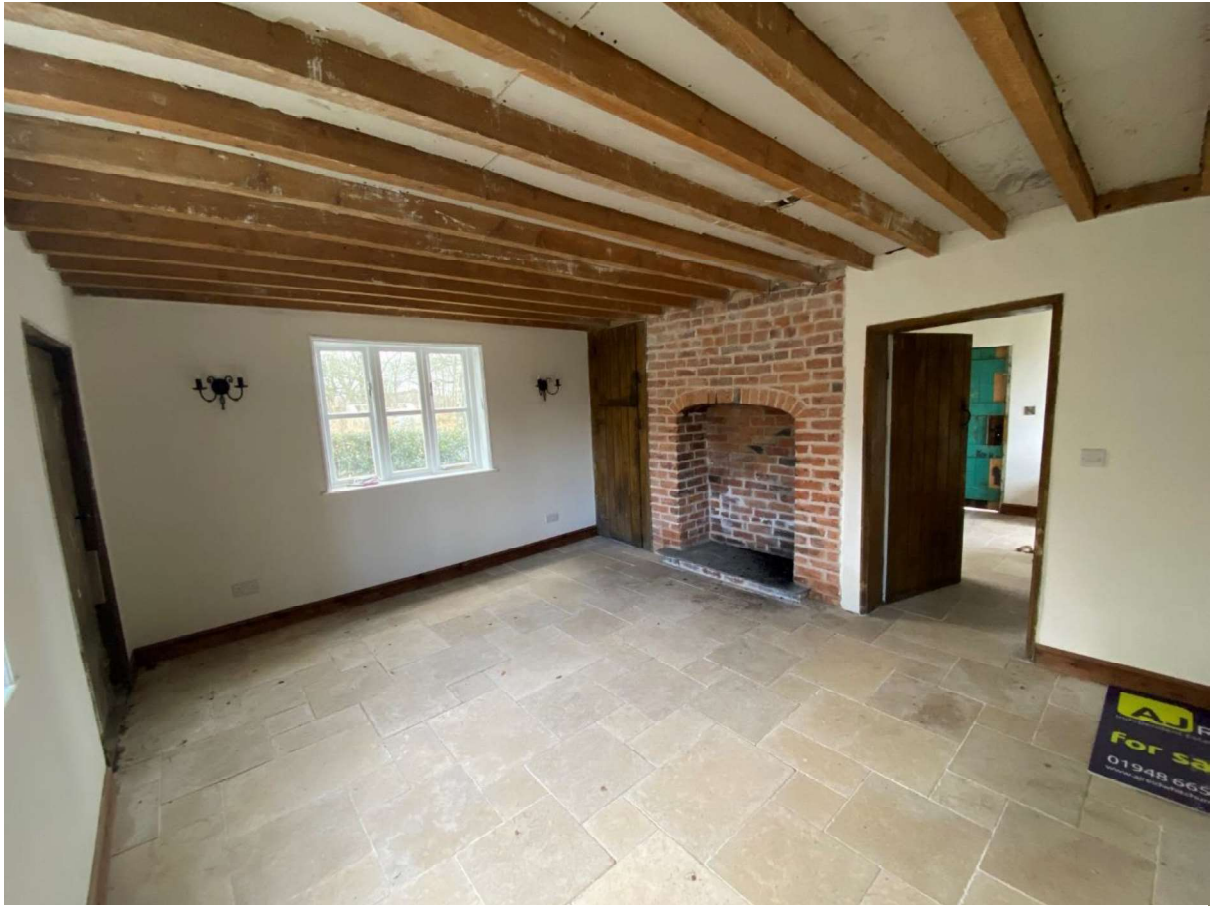
Figure 6: Main living space within the Site. The significant fireplace is visible, as is the newly installed skirting boards.
