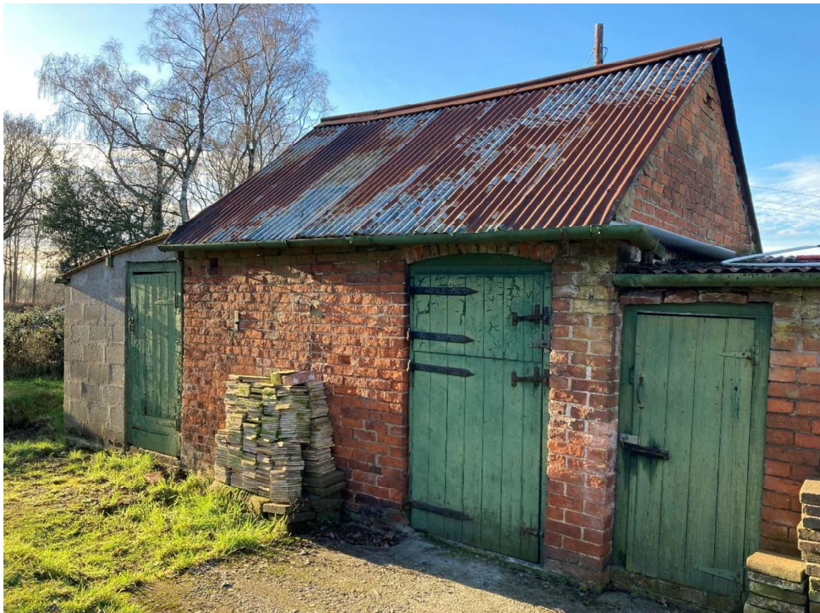
Figure 6: Former cow-pen, with breezeblock lean-to proposed for removal and adjoining brick store
