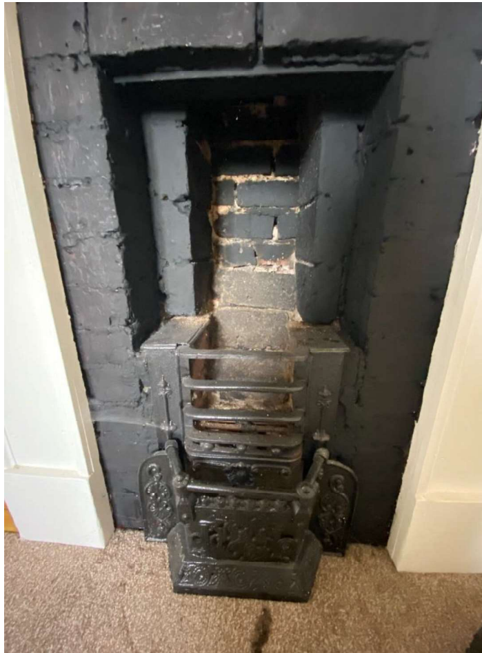
Figure 4: Historic fireplace surround in bedroom one.
