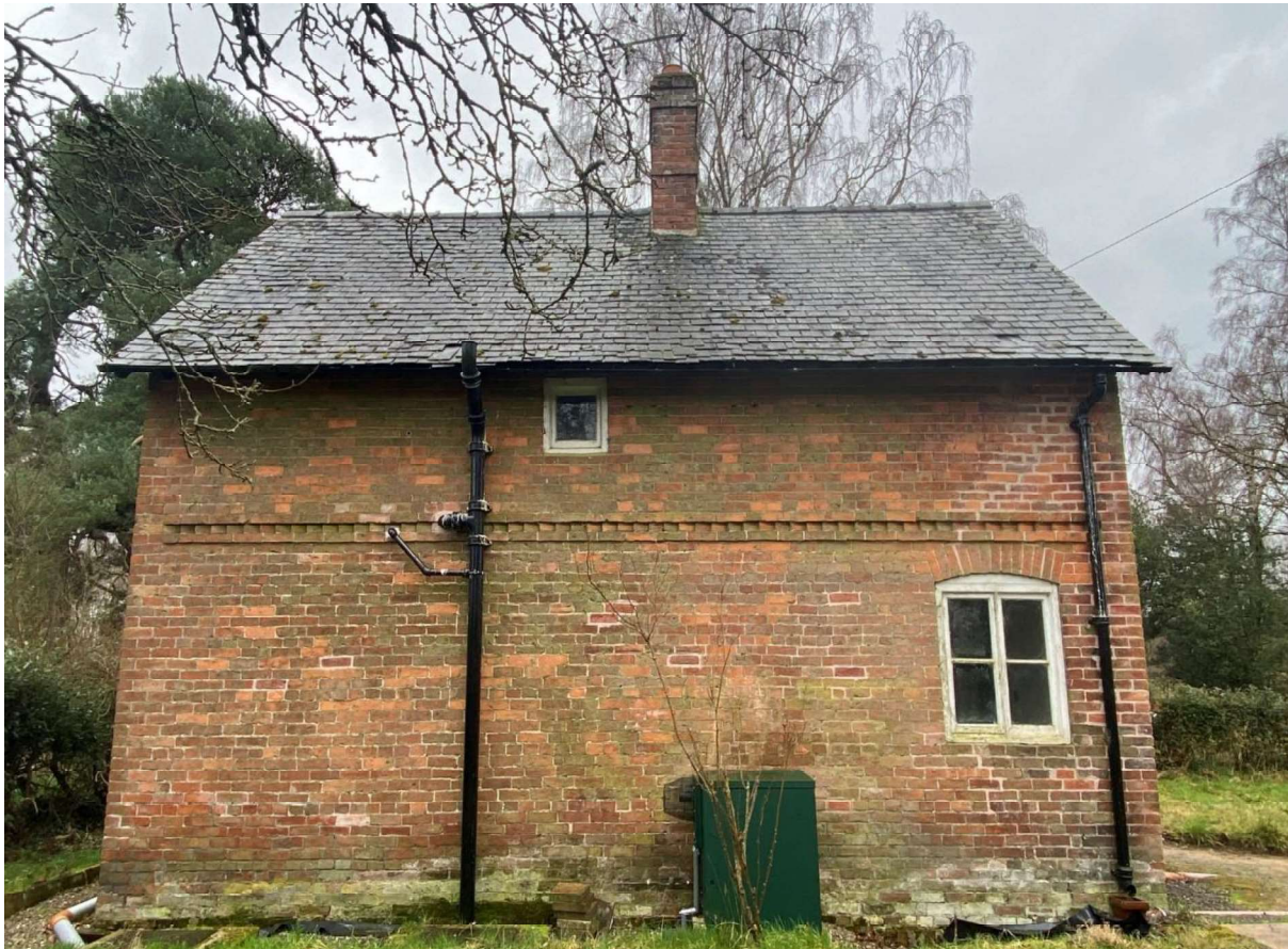
Figure 2: The northeast elevation of the Site. This Site features the architecturally interesting small, square window, as well as a portion of the dog toothed corbelling detail.
