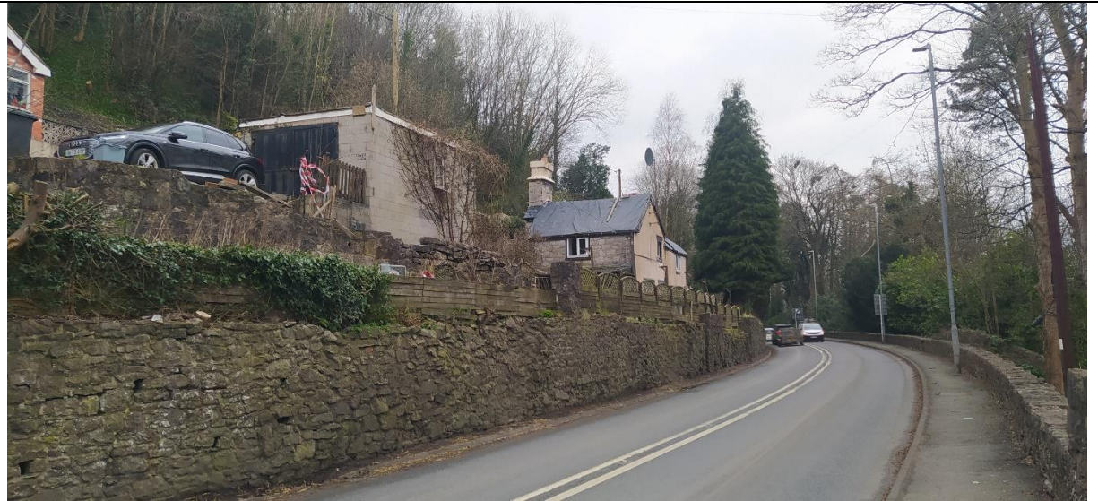
Photo 1 – shows the east and north-facing elevation of the garage and the dwelling
