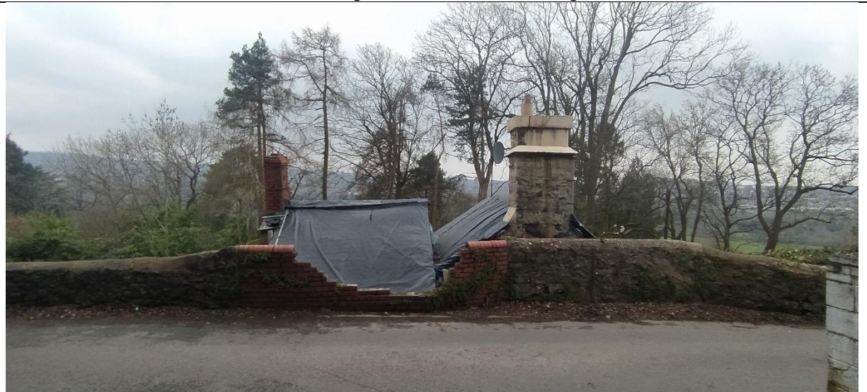
Photo 3 – shows south-facing roof of the dwelling
