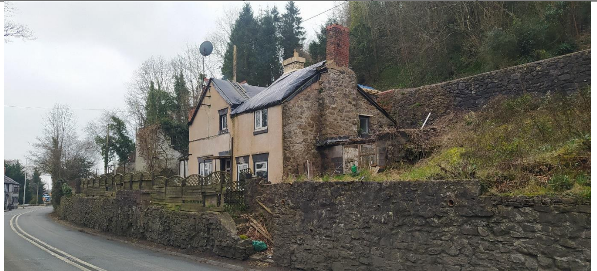
Photo 2 – shows the west and north-facing elevations of the dwelling
