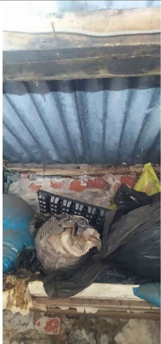
Photo 8 – shows the corrugated galvanised steel roof of part of the lean to
