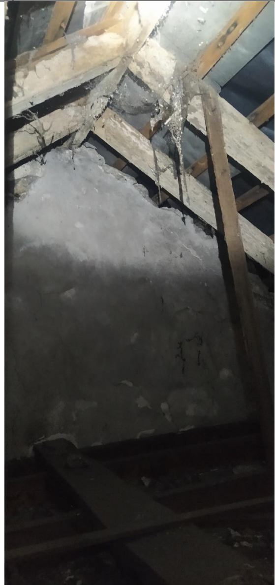
Photo 6 – shows the second 'cobwebby' roof void
