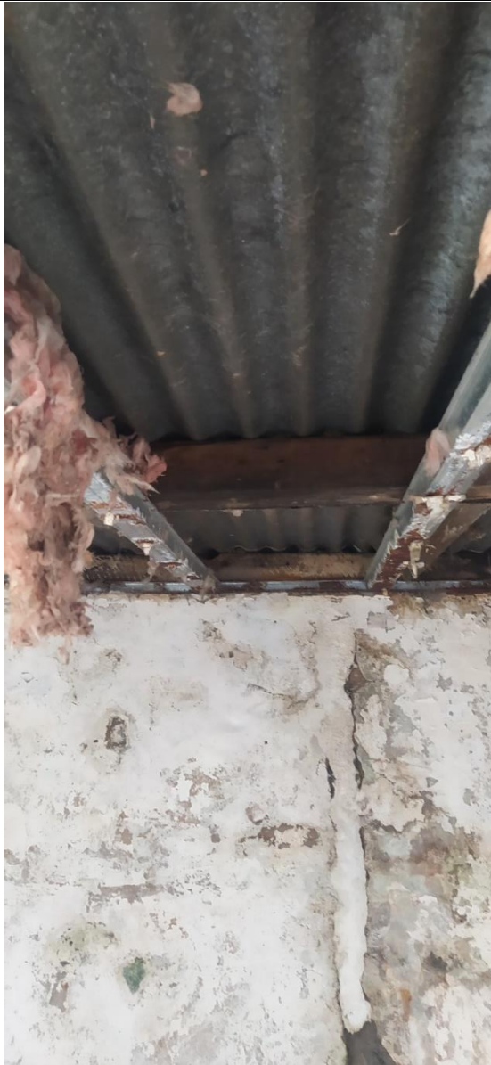
Photo 7 – shows the corrugated 'onduline' like material roof of part of the lean to
