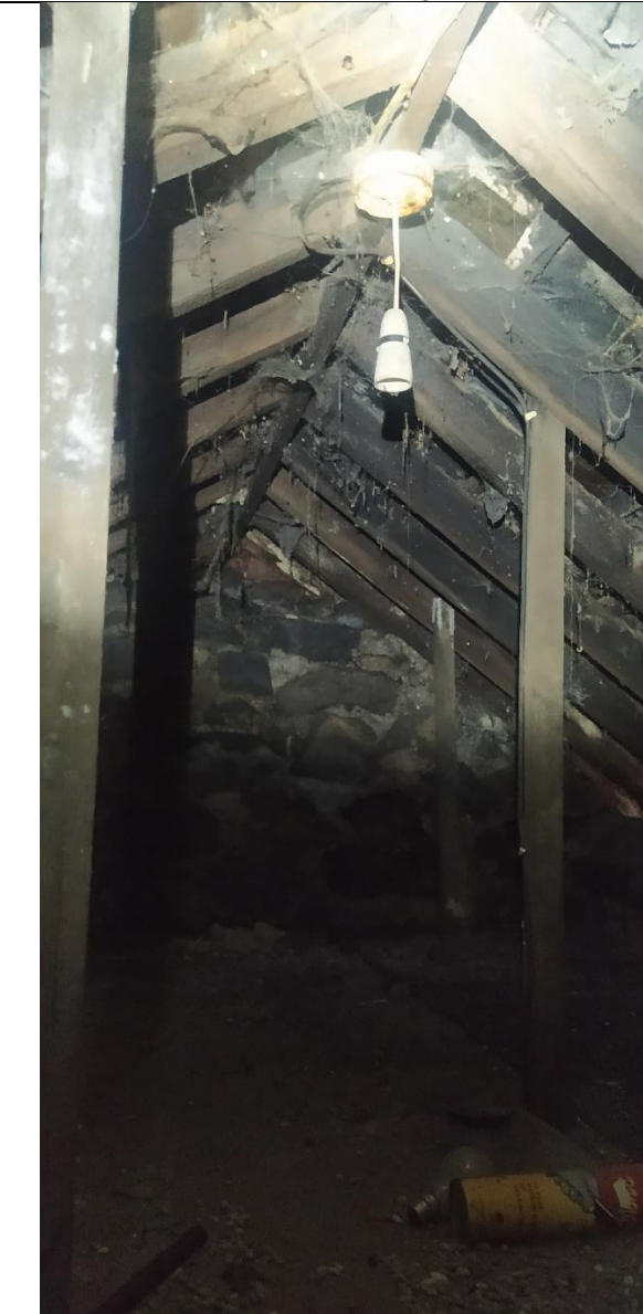
Photo 5 – shows one of the two 'cobwebby' roof voids
