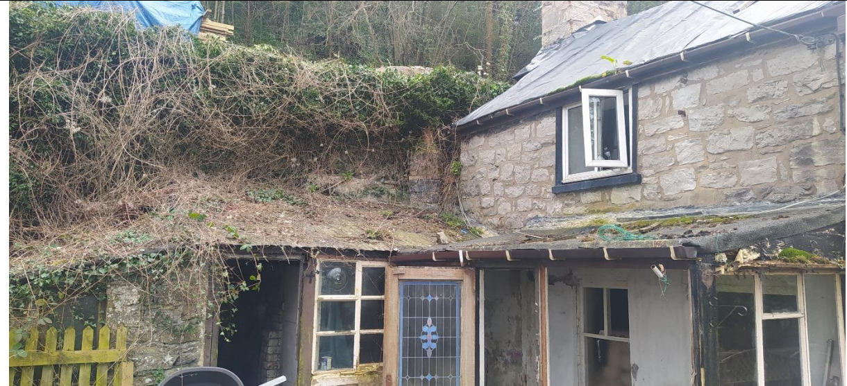
Photo 4 – shows the east-facing elevation of the dwelling with the lean-tos
