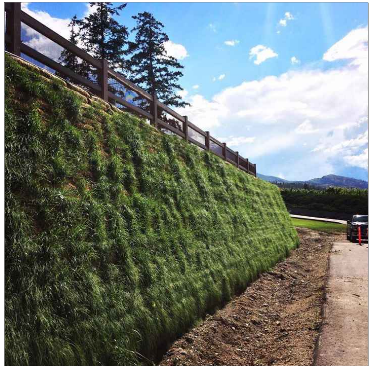
Typical vegetated wall after vegetation development
