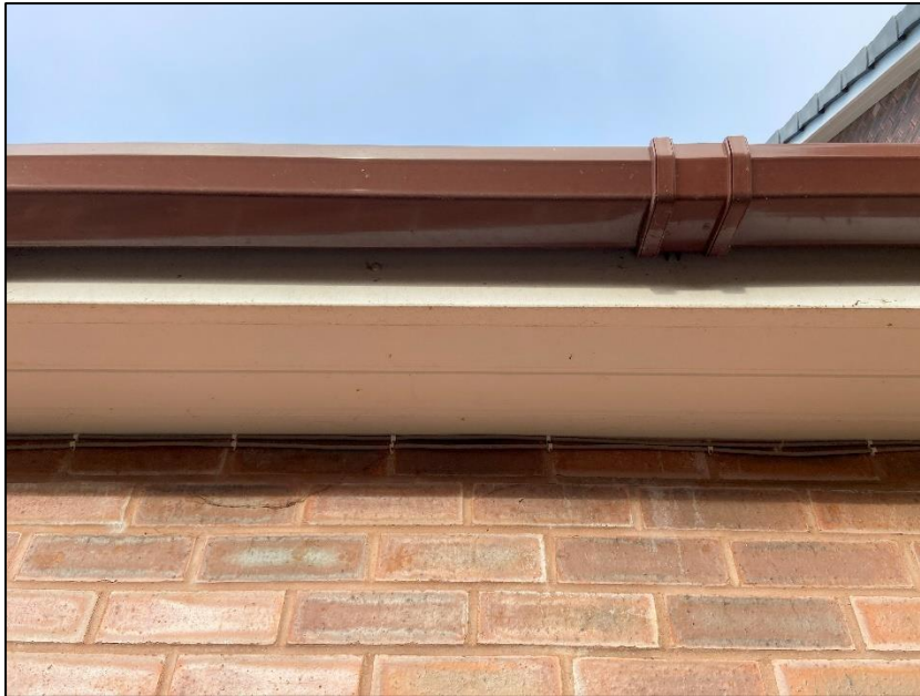
Photograph 11 showing uPVC soffit boards
