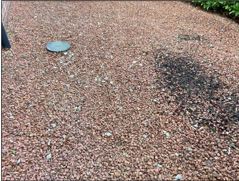
Photograph 4 showing the gravel pathway on site
