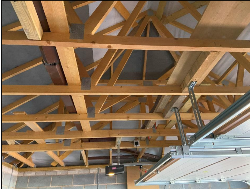
Photograph 13 showing the interior of the garage
