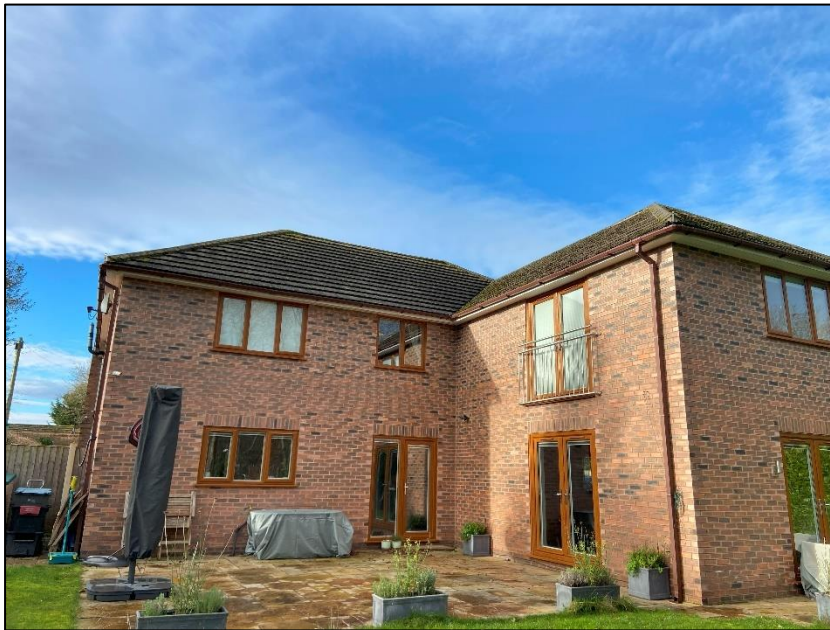
Photograph 8 showing the southeastern elevation of the building
