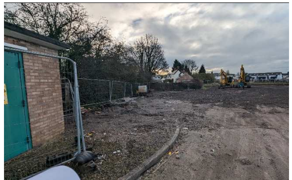
Photograph 4: View to south east of electricity sub-station, with garage and tarmac stripped. Photograph received by Coopers from Castlemead Group Limited on 31 st January 2024
