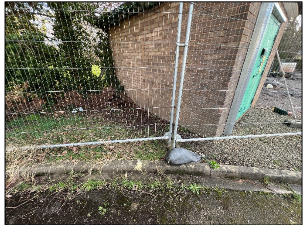
Photograph 2: North west side of electricity sub-station. Photograph taken by Coopers on 2 nd February 2024
