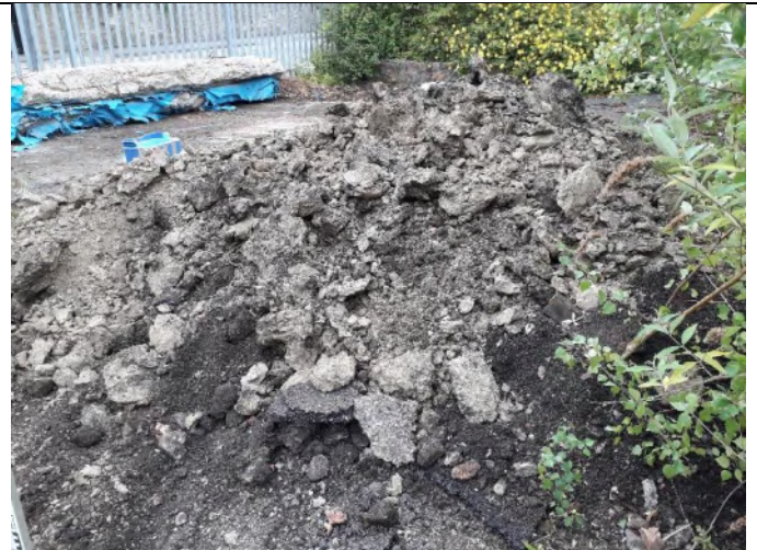
Trial Pit 03: Overview of excavated soils
