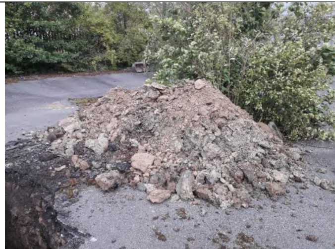
Trial Pit 04: Overview of excavated soils
