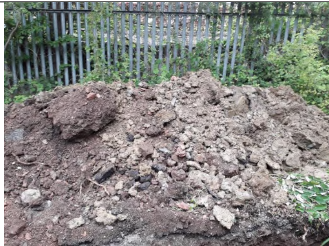
Trial Pit 01: Overview of excavated soils
