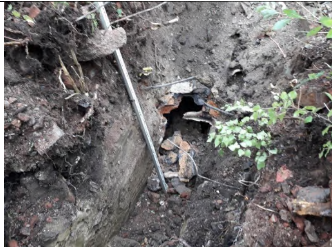
Trial Pit 10: Overview of excavated soils
