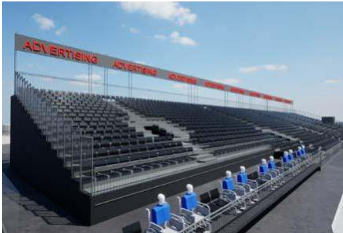
View of Stand from North -West Corner
