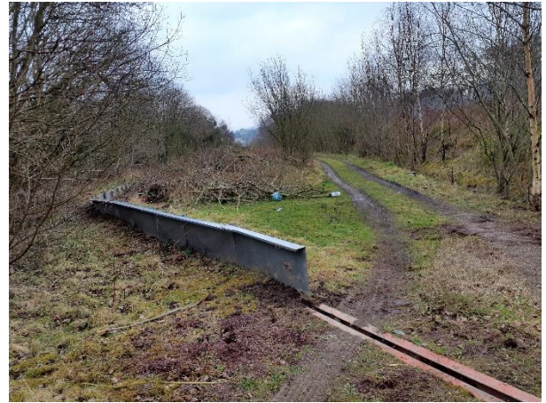
FIGURE 4.7: AMPHIBIAN EXCLUSION GRILLE AT THE WESTERN END OF THE FENCING
