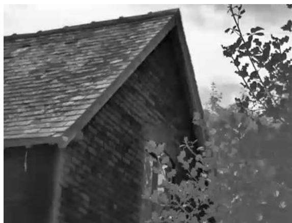
P16: 2 nd thermal imaging camera view (SE gable)
