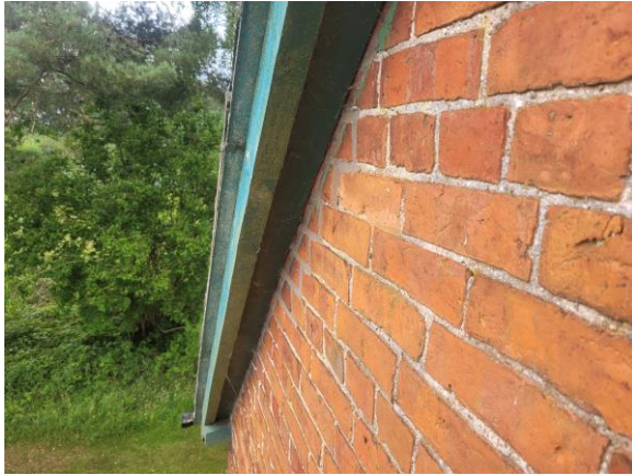
P7: Example of the close-fitting gable rafters
