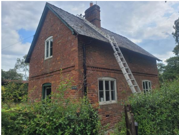
P1: NW (gable) + SW (side) elevations: looking E
