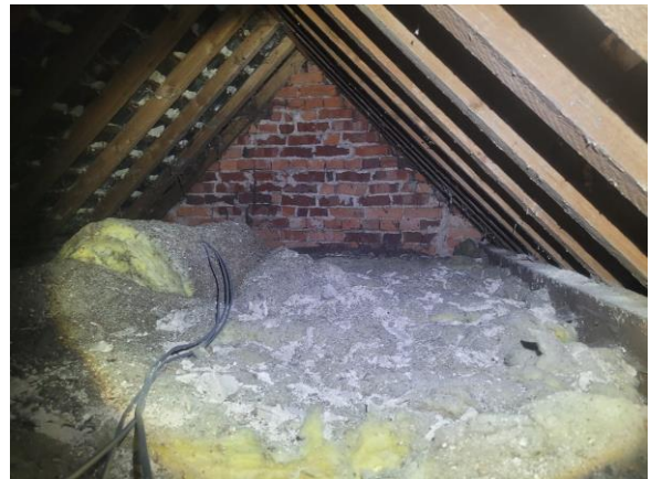
P4: N loft: viewed from the S end, looking NW
