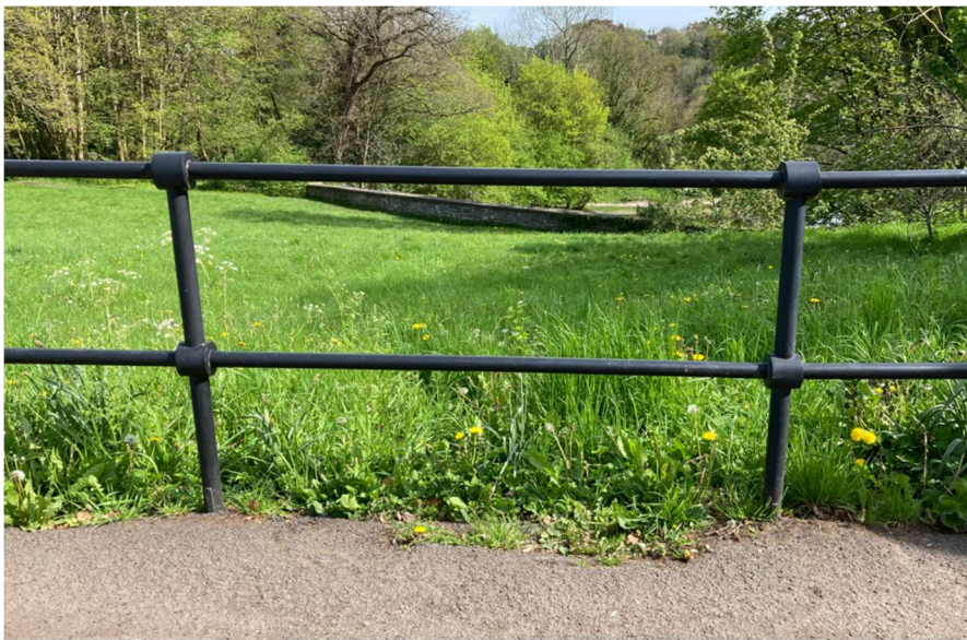
Figure 2 - Photograph showing the existing railings, with the parapet wall above Chirk Tunnel's south portal visible in the background.
