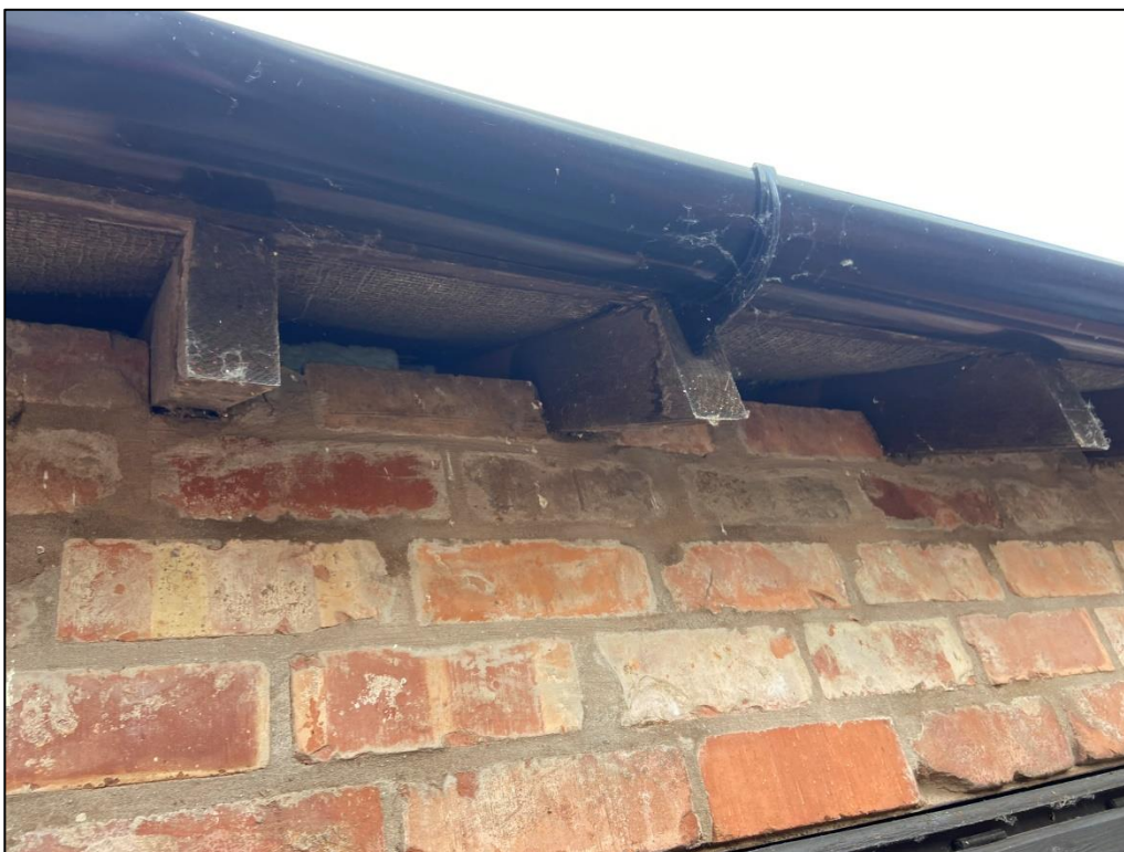
Plate 10 – Further character of the open eaves
