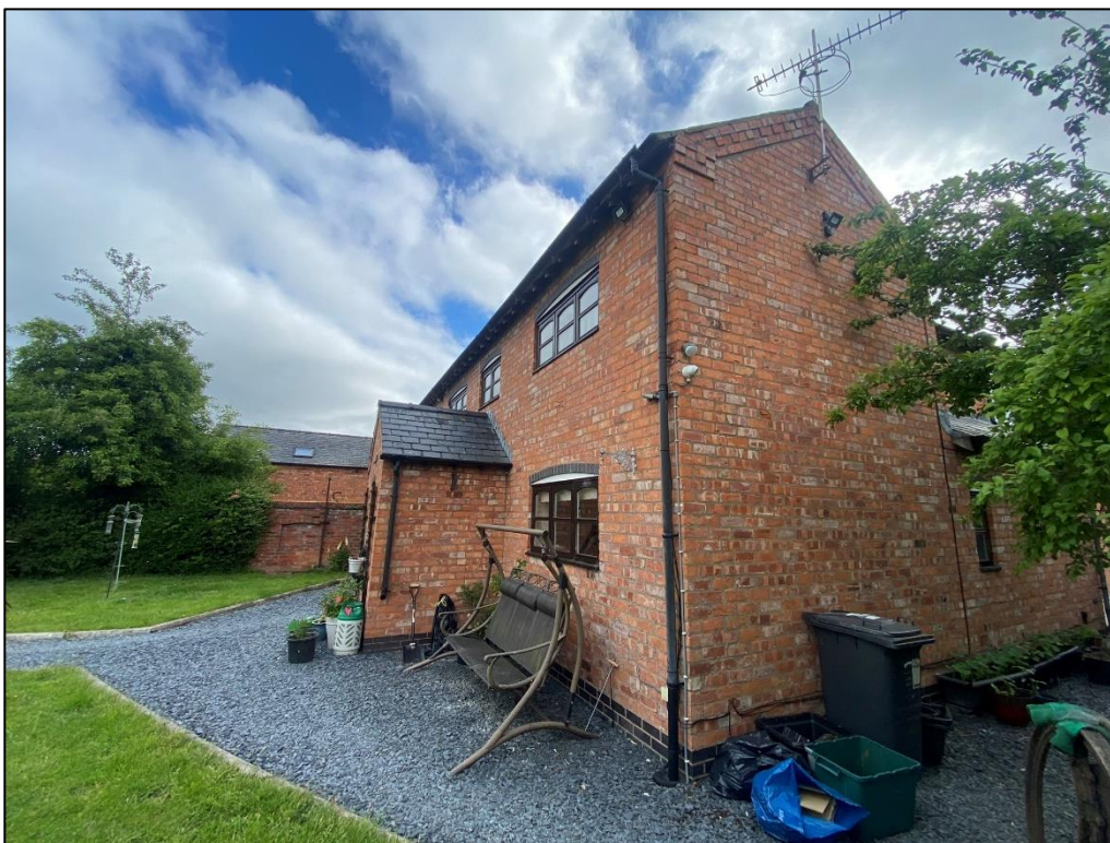
Plate 5 – Character of the southern gable elevation of the dwelling
