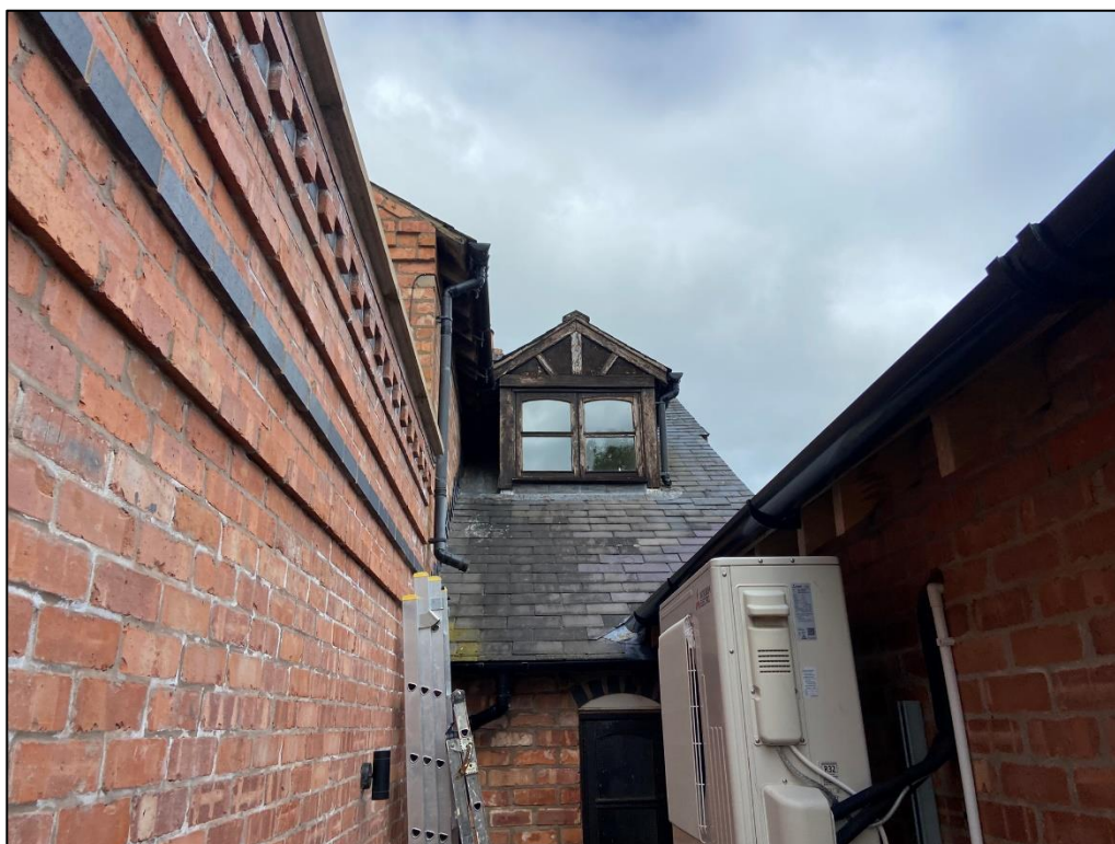
Plate 8 – Character of a dormer window located to the north of the dwelling
