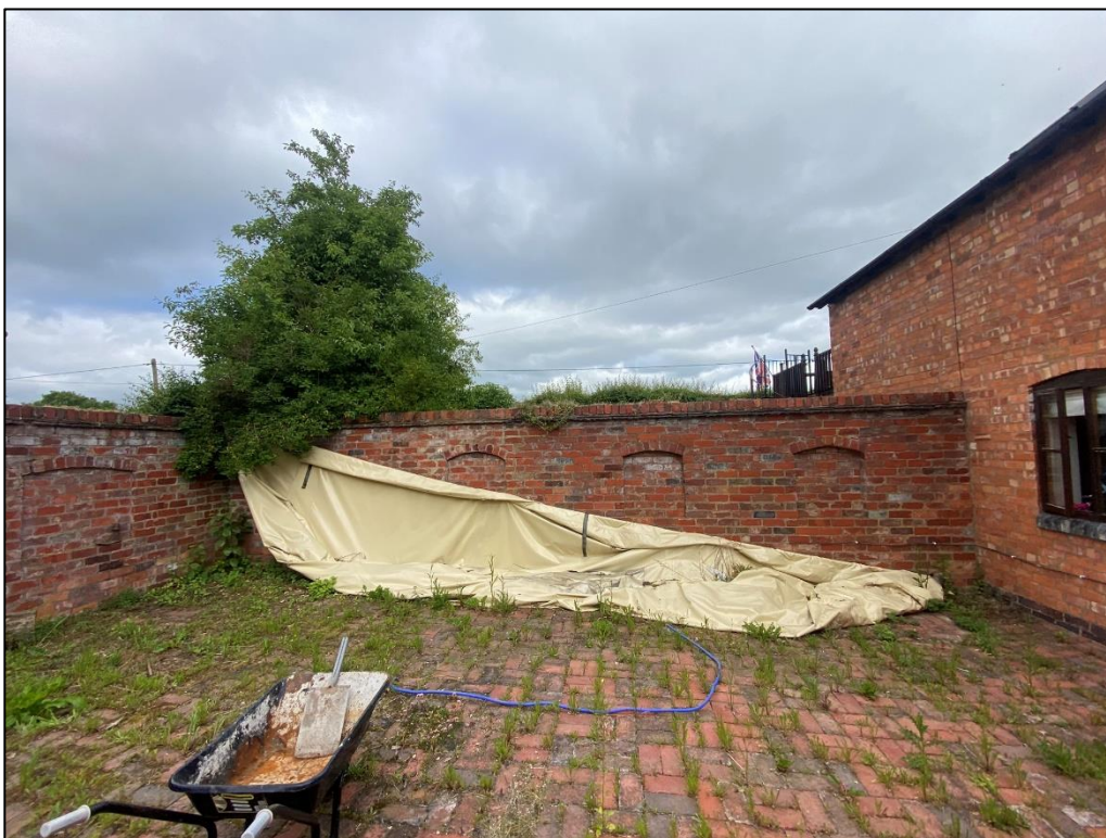
Plate 4 – Character of the courtyard where works are proposed to occur
