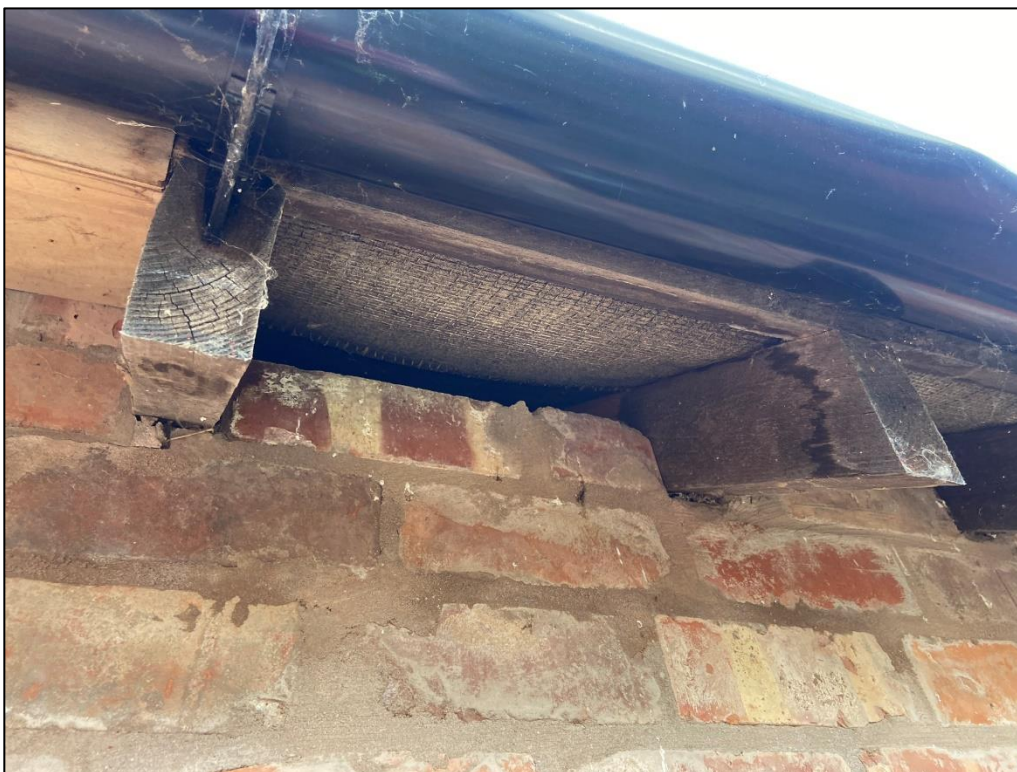
Plate 9 – Open eaves located at the adjoining portion of the building
