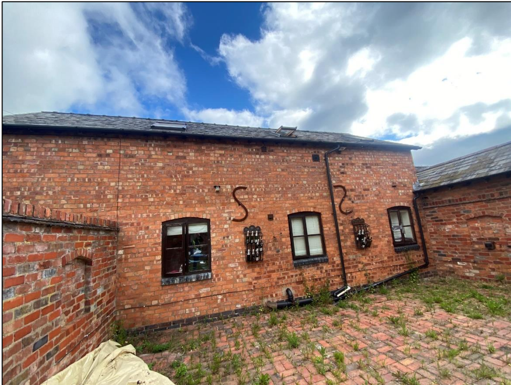
Plate 3 – Character of the northerly adjoining building
