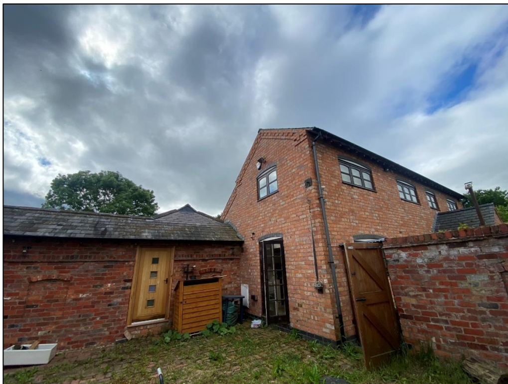
Plate 1 – Character of the northern gable elevation of the dwelling
