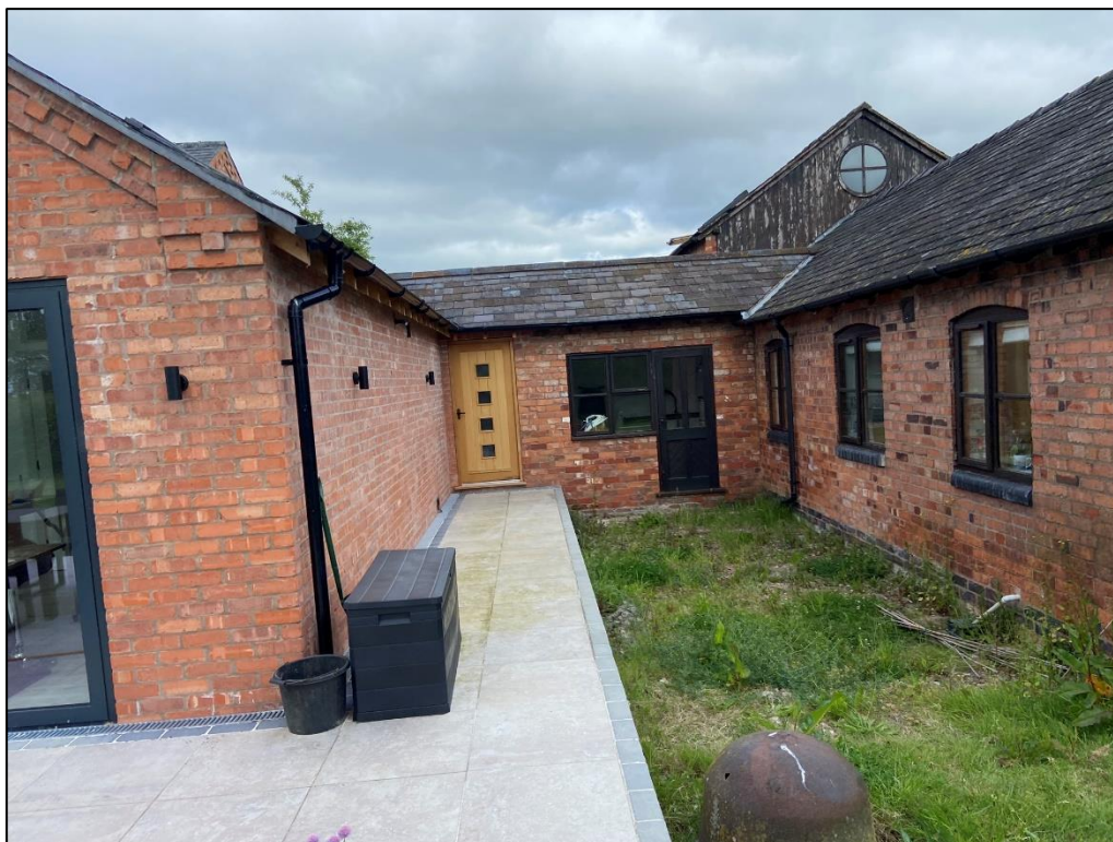
Plate 12 – Further character of the eastern elevation of the adjoining section of the building
