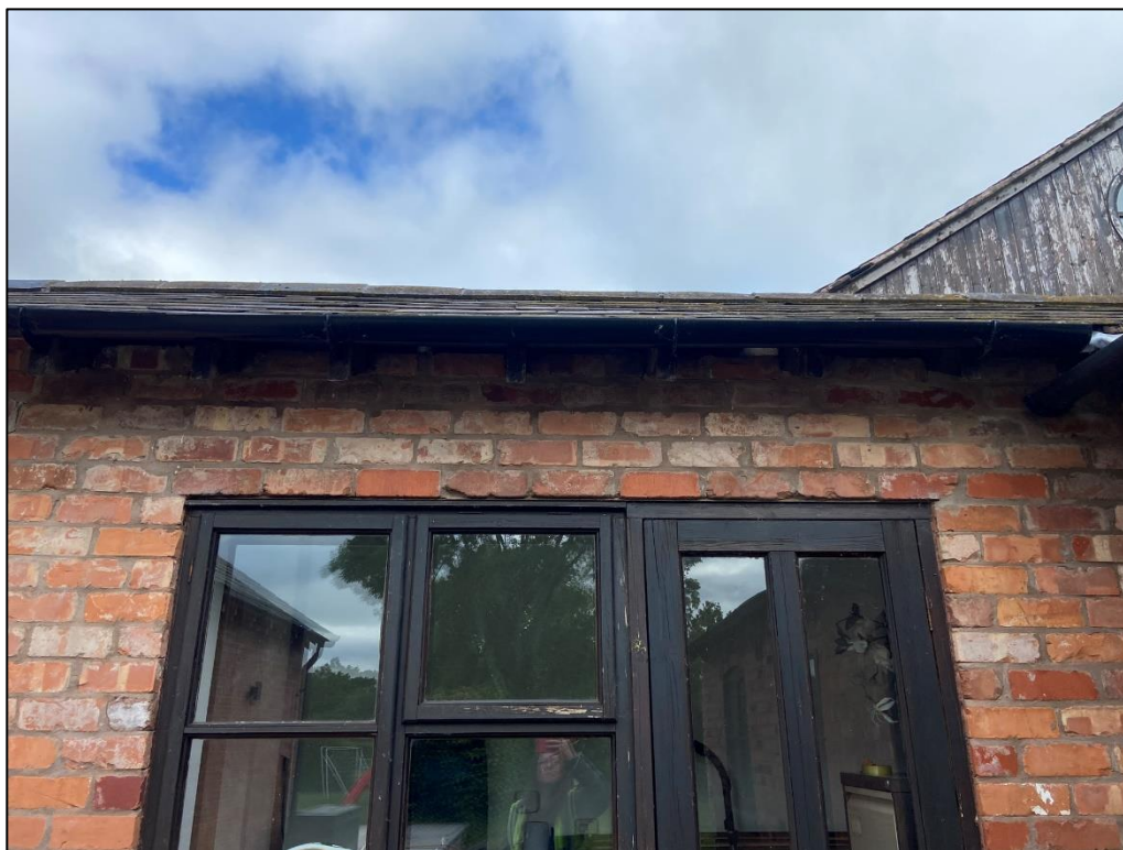
Plate 11 – Character of the eastern elevation of the adjoining section of the building
