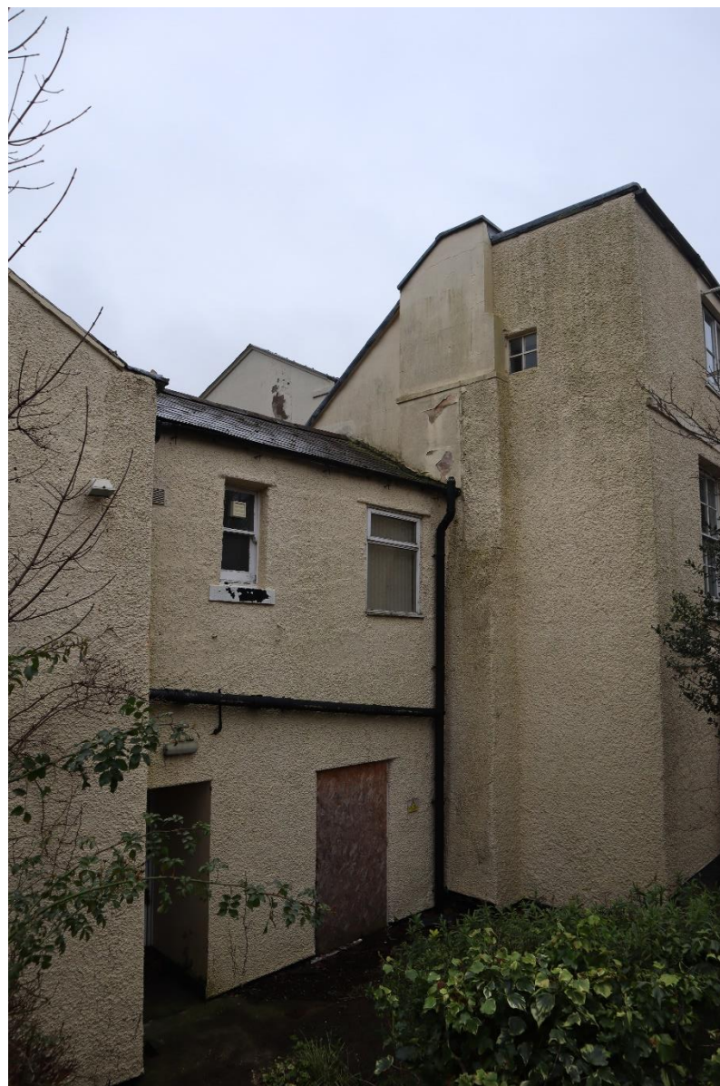
Figure 23 – Rear of 24 Chester Street
