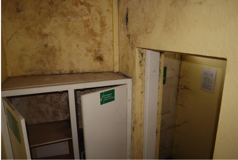
Figure 197 – Stairway of 24 Chester Street
