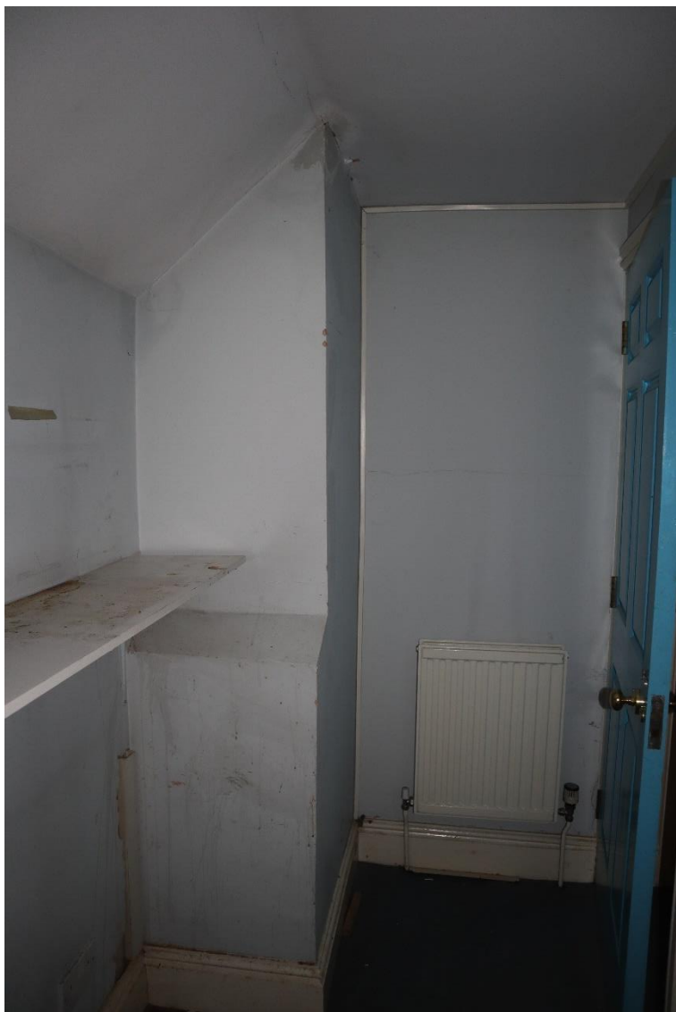
Figure 163 – Rear second floor rooms of 23 Chester Street
