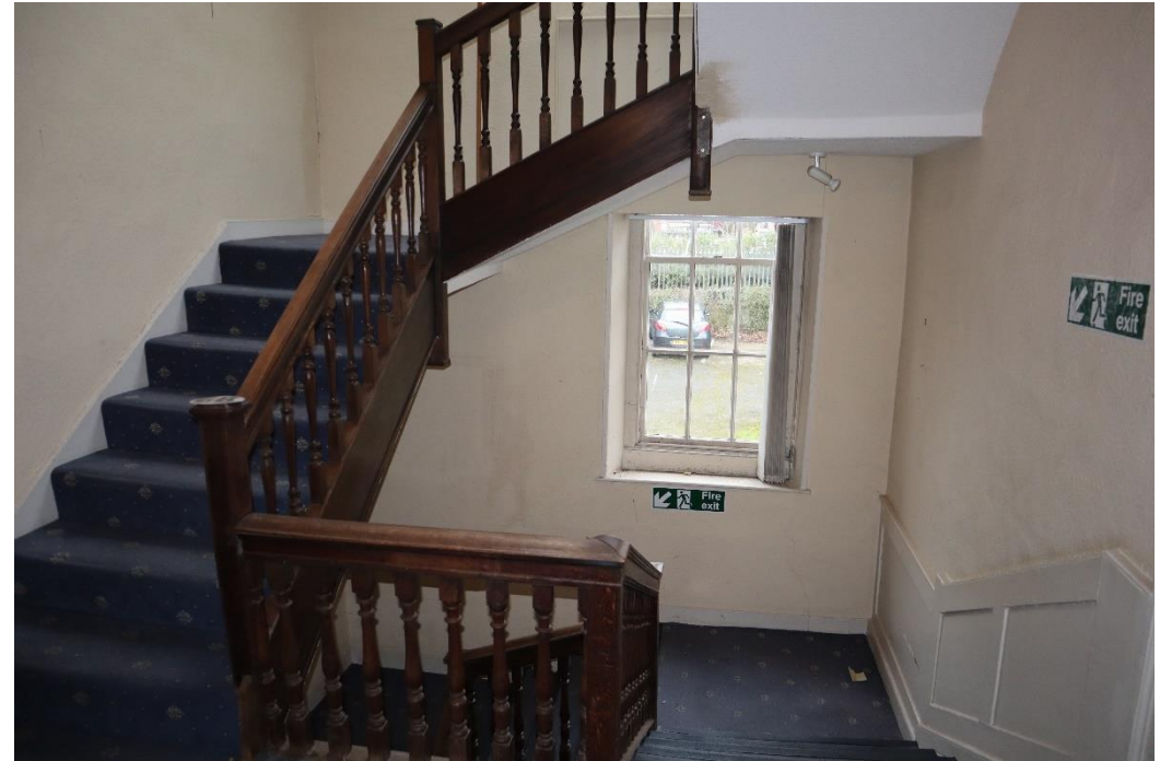
Figure 93 – First floor stairwell of 23 Chester Street
