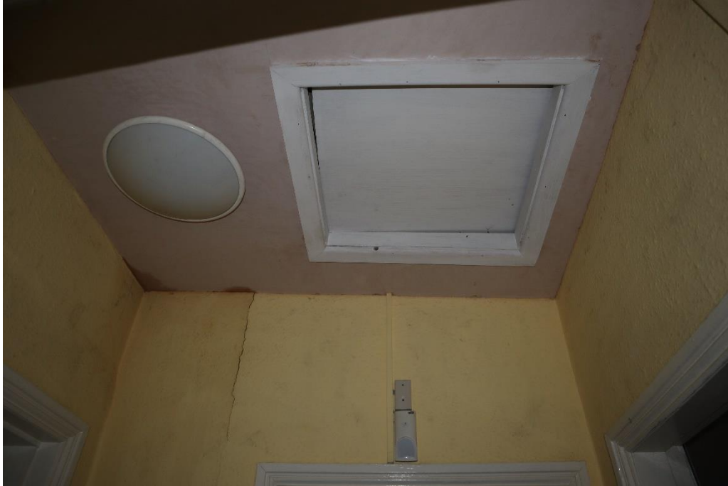
Figure 215 – Loft hatch of 24 Chester Street
