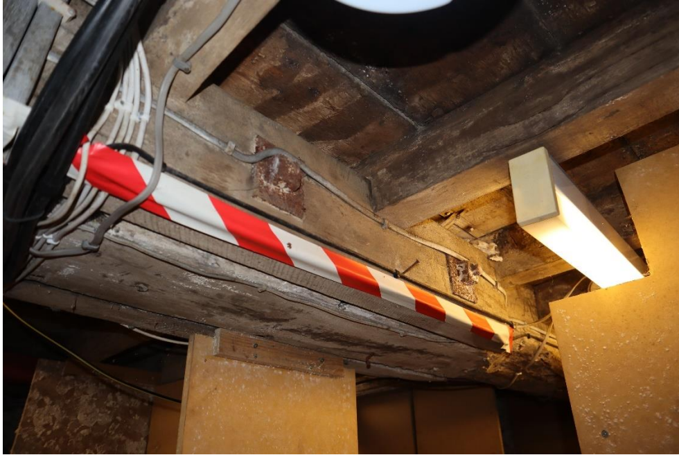
Figure 61 – Basement of 23 Chester Street
