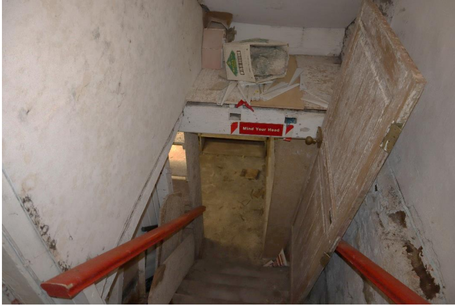
Figure 49 – Basement of 23 Chester Street
