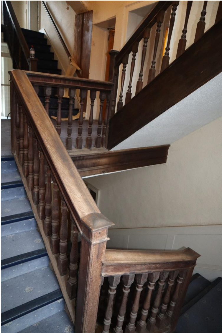
Figure 92 – First floor stairwell of 23 Chester Street
