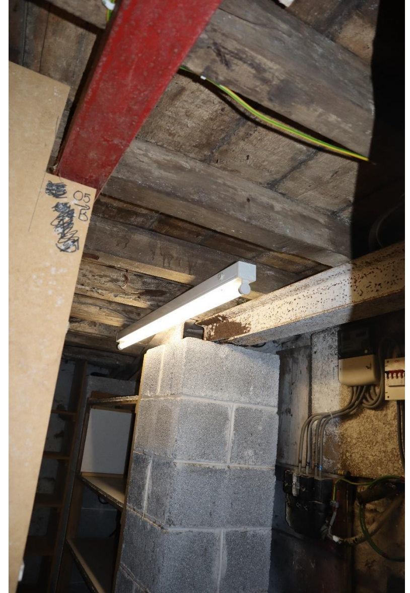
Figure 58 – Basement of 23 Chester Street
