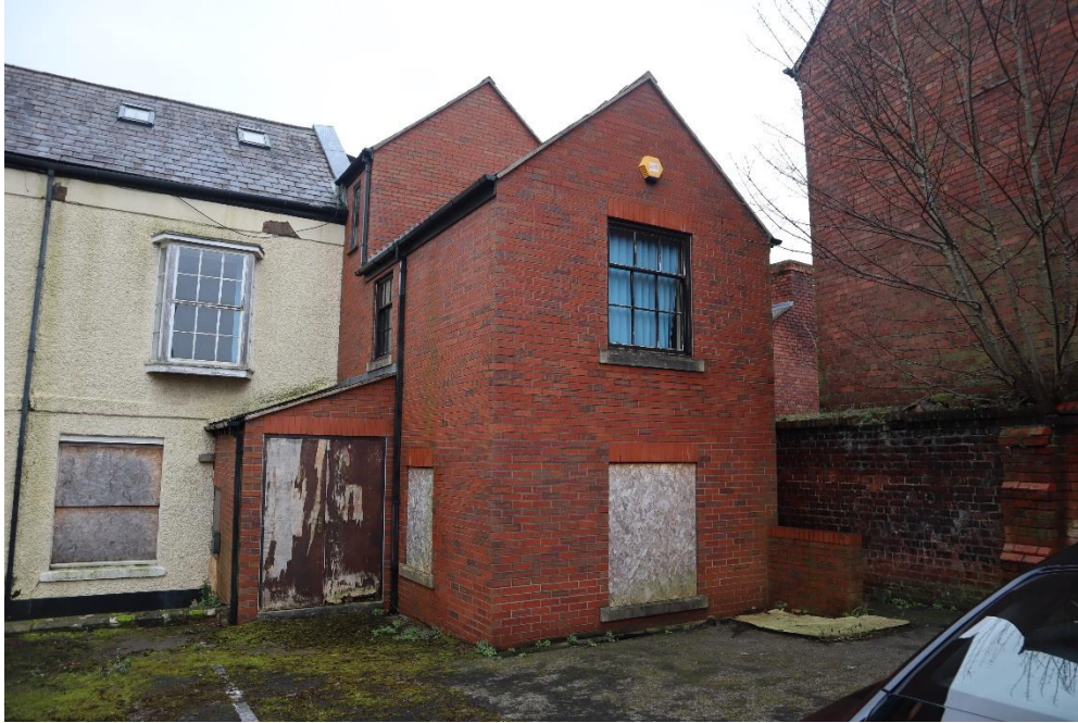
Figure 16 – Rear of 23 Chester Street
