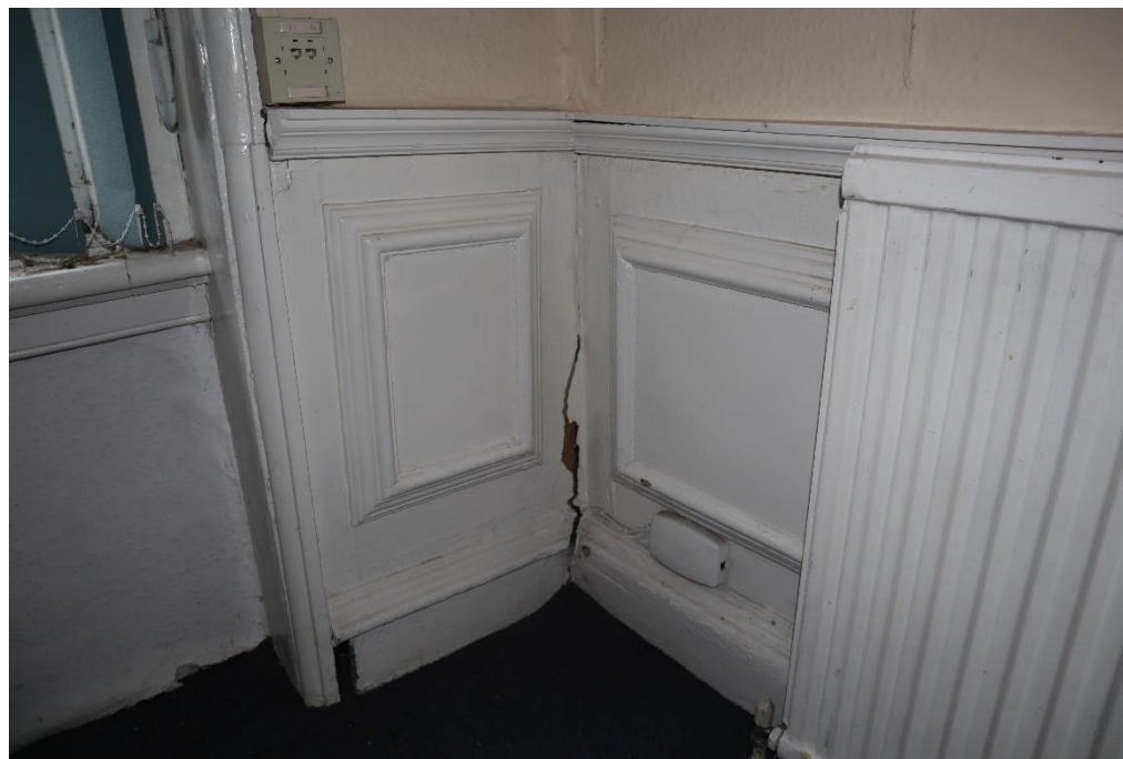
Figure 135 – Room 12 of 23 Chester Street
