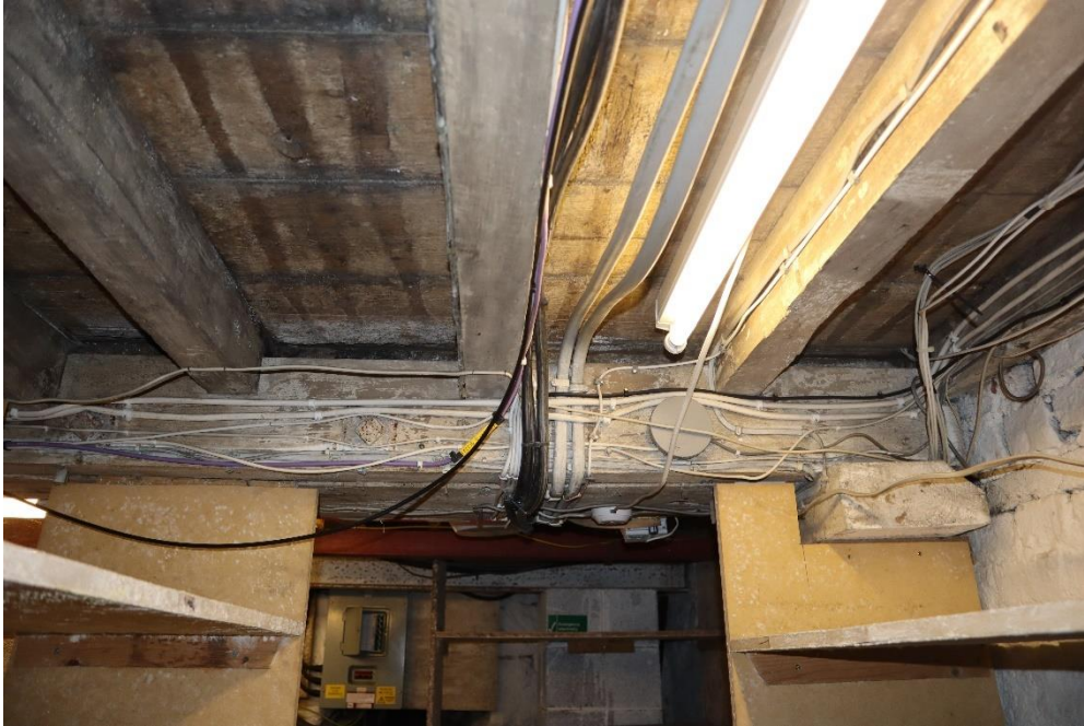
Figure 57 – Basement of 23 Chester Street
