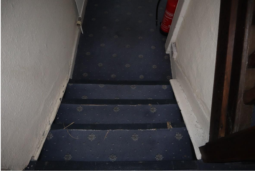
Figure 96 – First floor stairwell of 23 Chester Street
