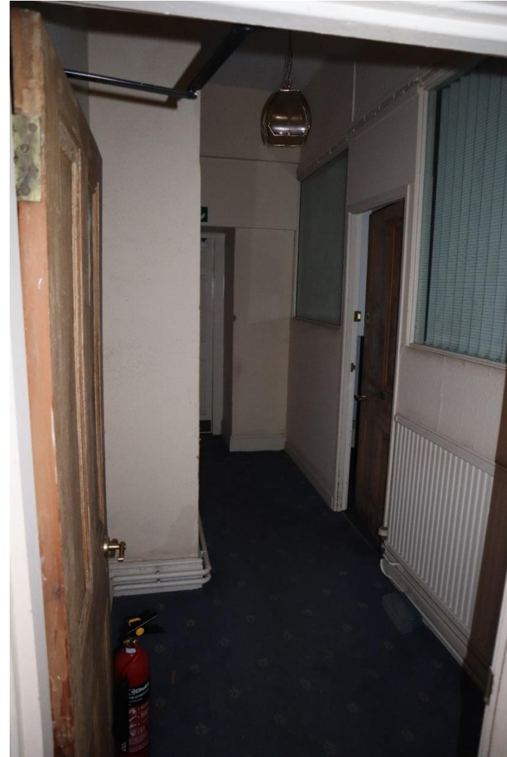
Figure 40 – Rear corridor to room 2 of 23 Chester Street
