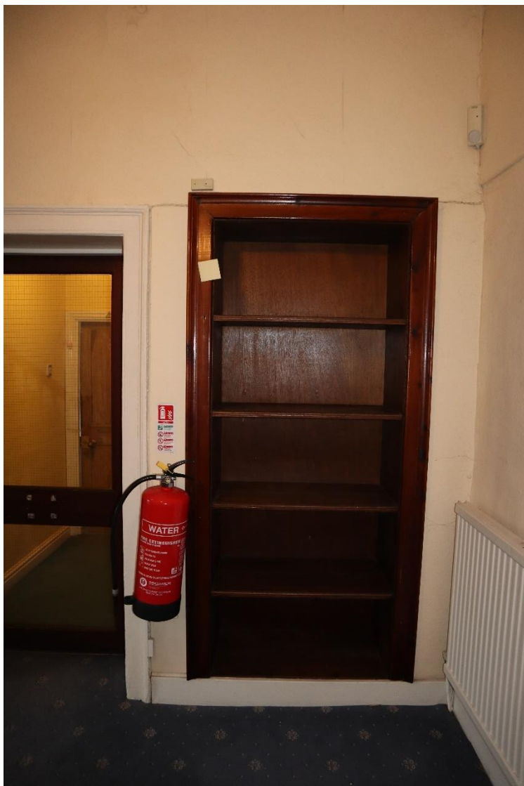
Figure 94 – First floor stairwell of 23 Chester Street
