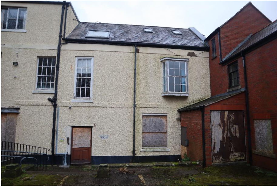
Figure 18 – Rear of 23 Chester Street
