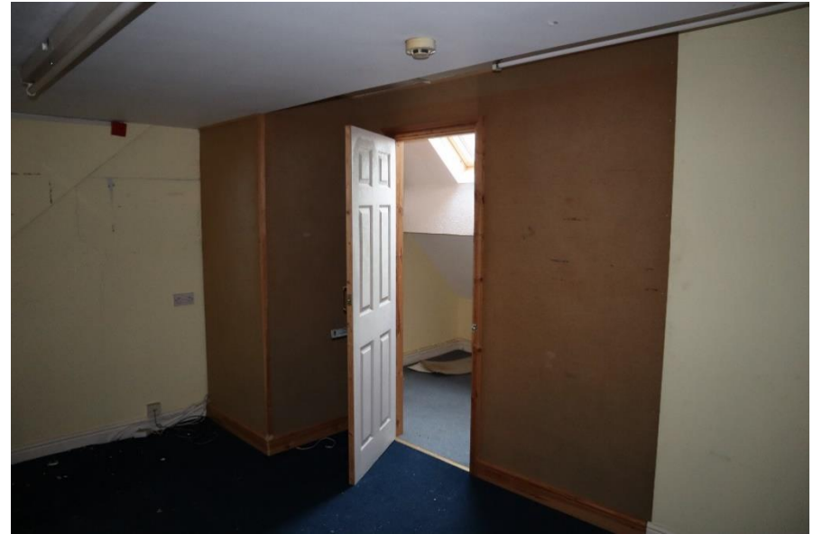
Figure 166 – Rear second floor rooms of 23 Chester Street
