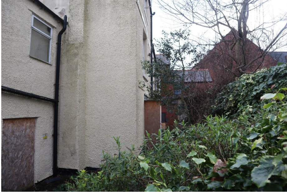
Figure 26 – Rear of 24 Chester Street
