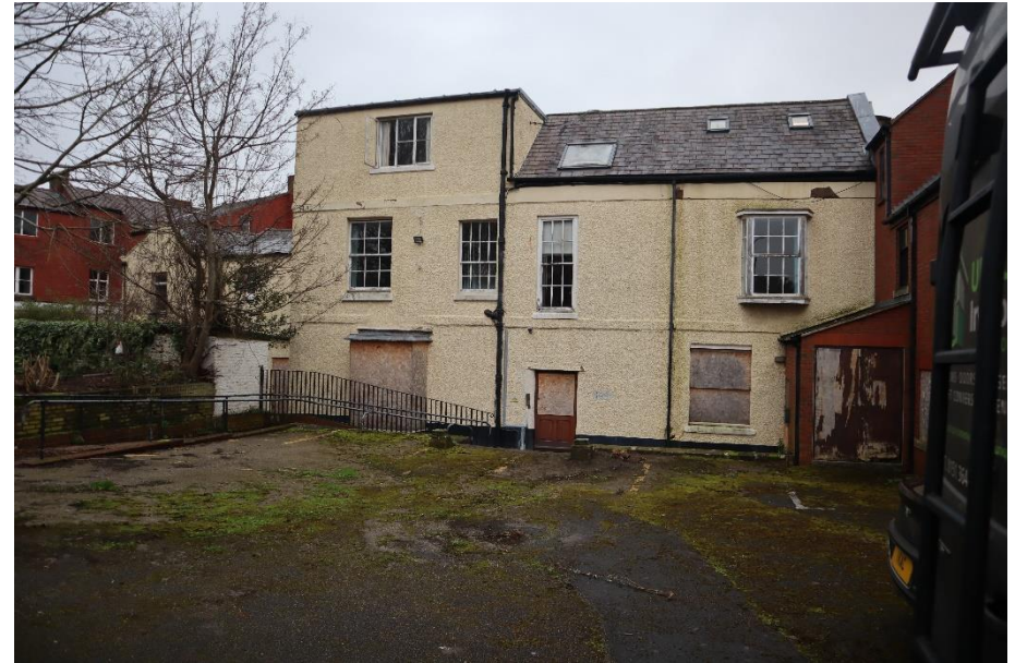
Figure 19 – Rear of 23 Chester Street
