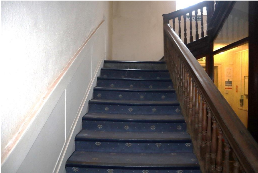
Figure 90 – Ground floor stairwell 23 Chester Street
