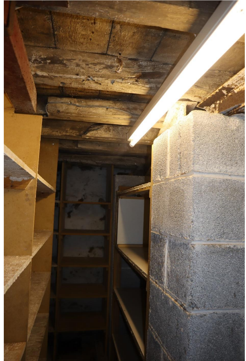
Figure 62 – Basement of 23 Chester Street
