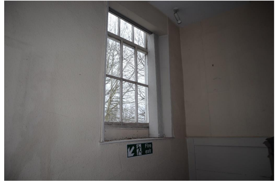
Figure 91 – First floor stairwell of 23 Chester Street
