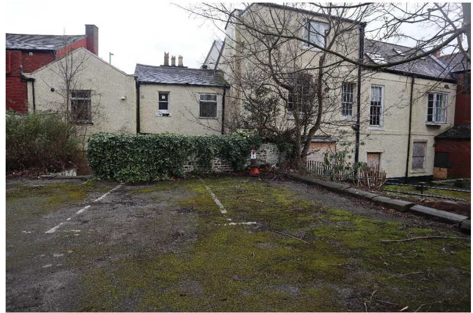
Figure 29 – Rear of 24 Chester Street
