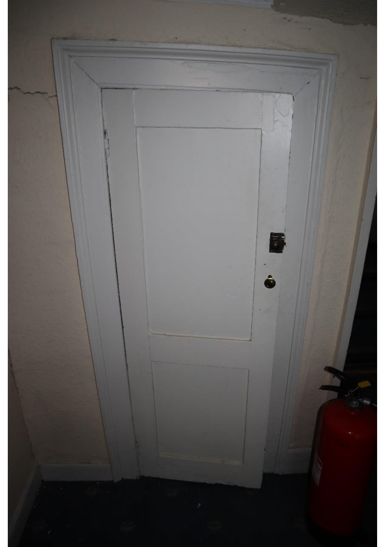
Figure 97 – First floor stairwell of 23 Chester Street
