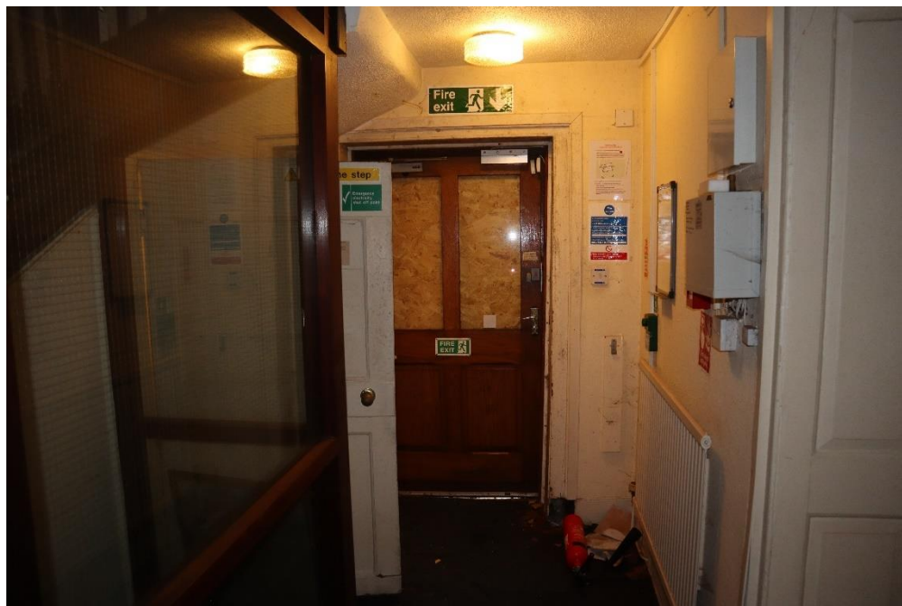
Figure 47 – Ground floor stairwell of 23 Chester Street
