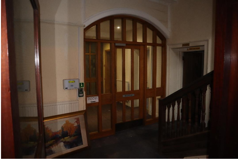
Figure 63 – Ground floor stairwell of 23 Chester Street
