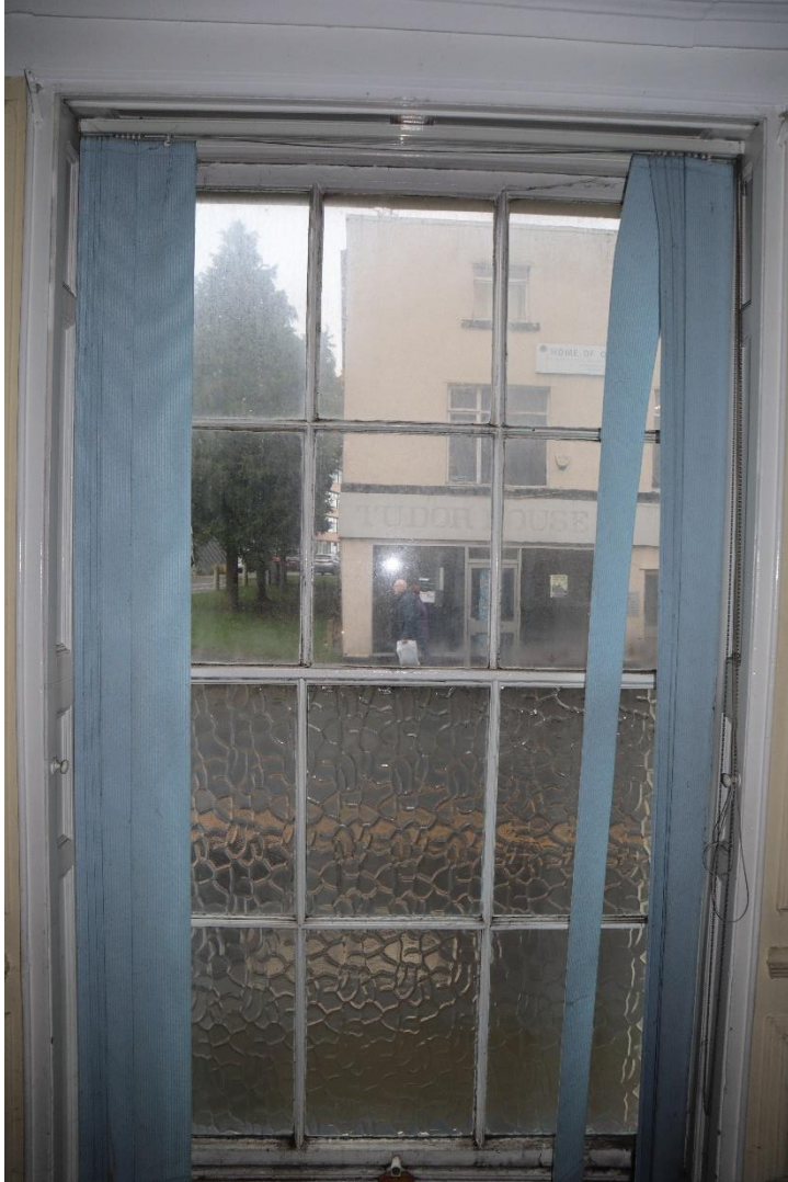
Figure 88 – Room 4 of 23 Chester Street
