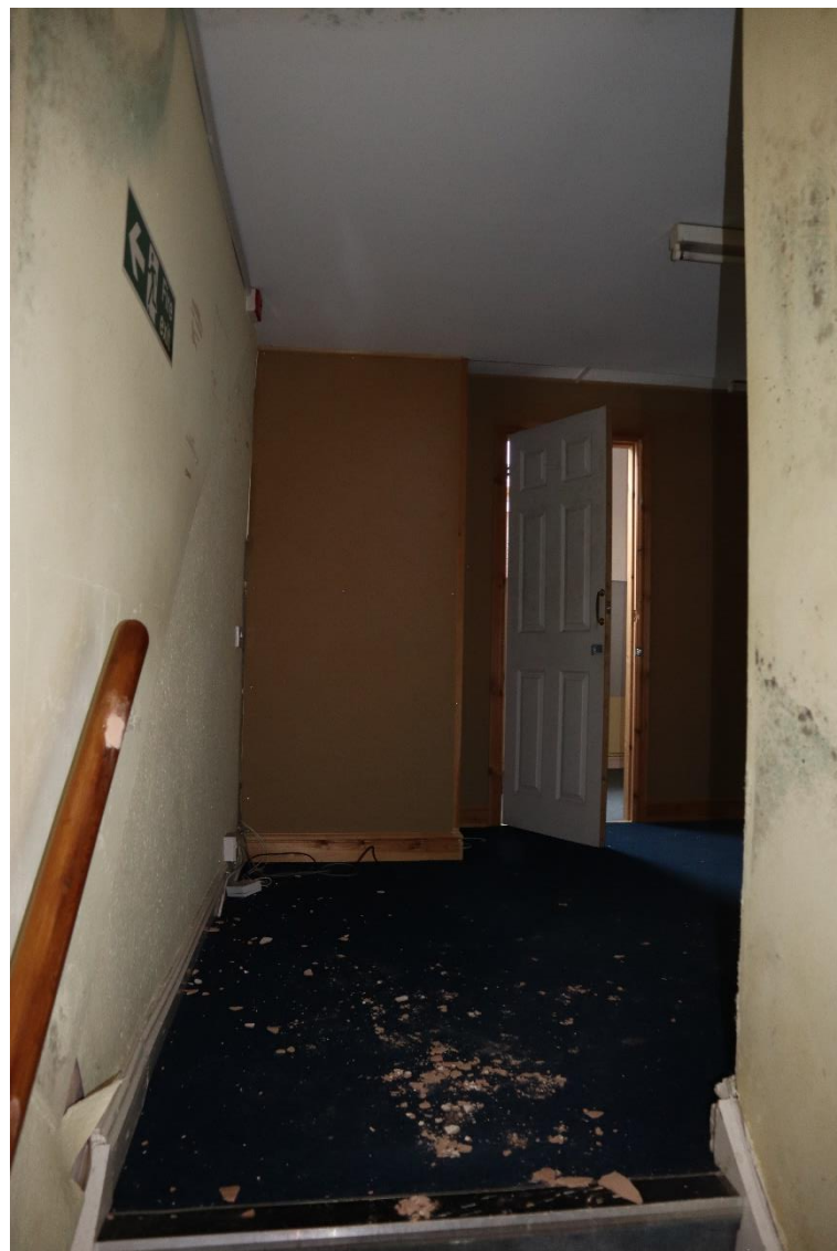
Figure 164 – Rear second floor rooms of 23 Chester Street
