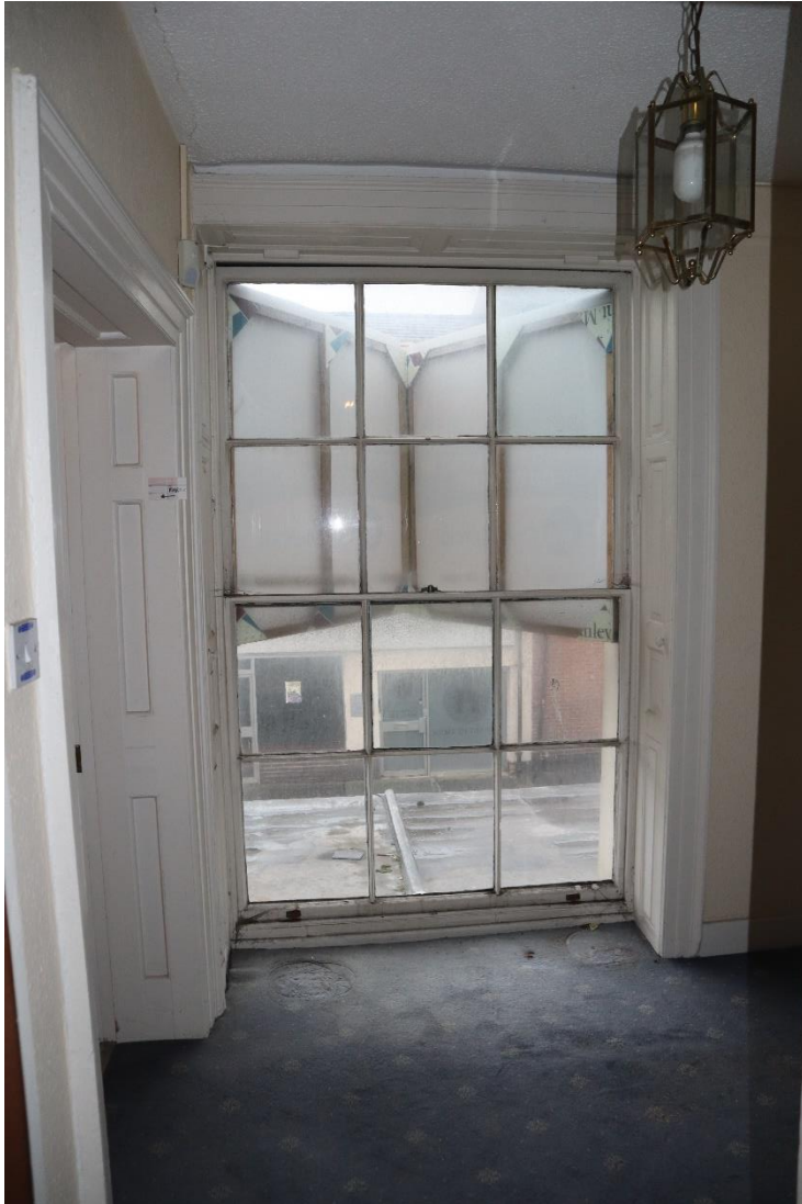
Figure 98 – First floor stairwell of 23 Chester Street
