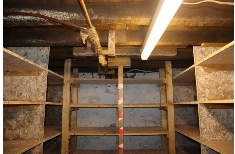
Figure 60 – Basement of 23 Chester Street
