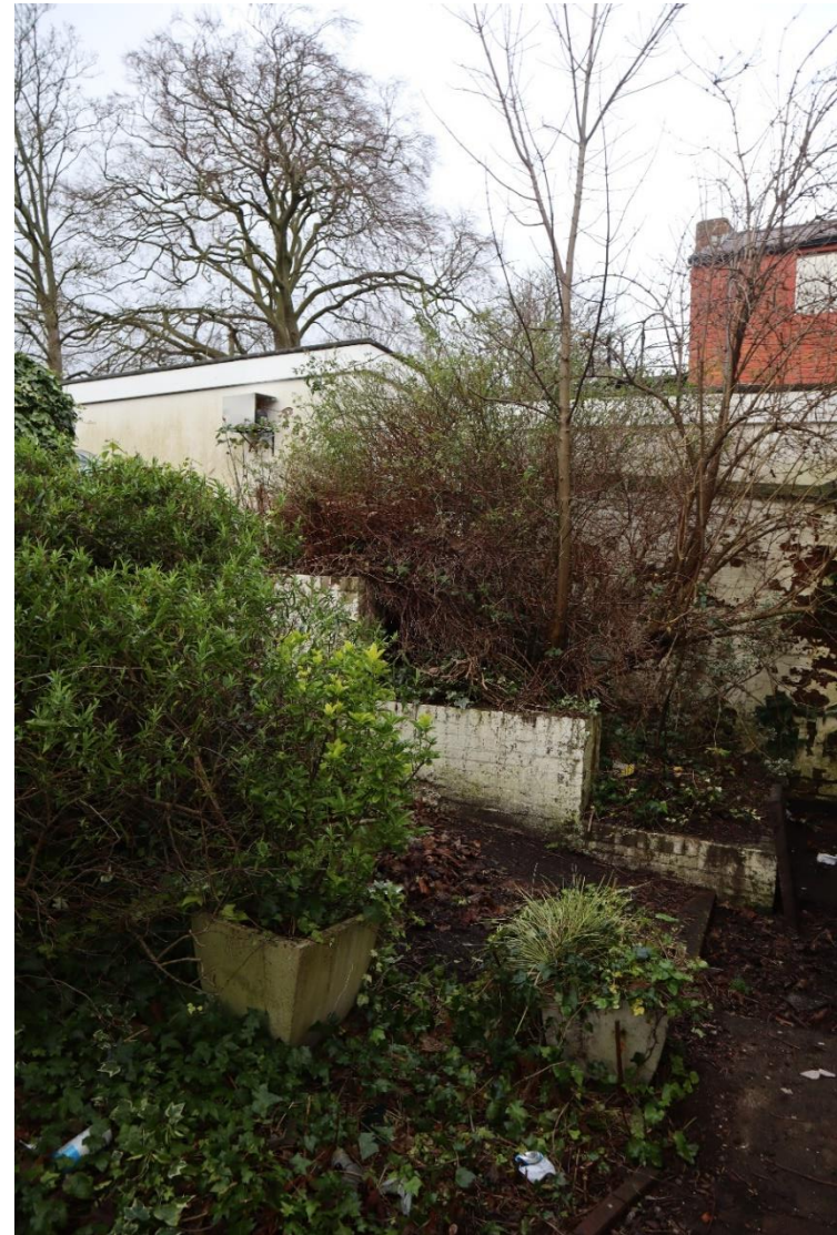
Figure 25 – Rear of 24 Chester Street
