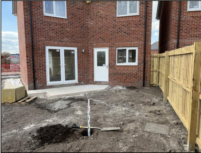
Photographs 4 & 5: Showing the depth of the inert cover and location of the validation hole within the rear garden of Plot 350 and the depth of inert cover achieved. Photographs taken 25 th April 2022.
