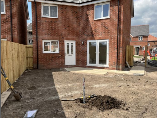
Photographs 1 & 2: Showing the depth of the inert cover and location of the validation hole within the rear garden of Plot 349 and the depth of inert cover achieved. Photographs taken 25 th April 2022.
