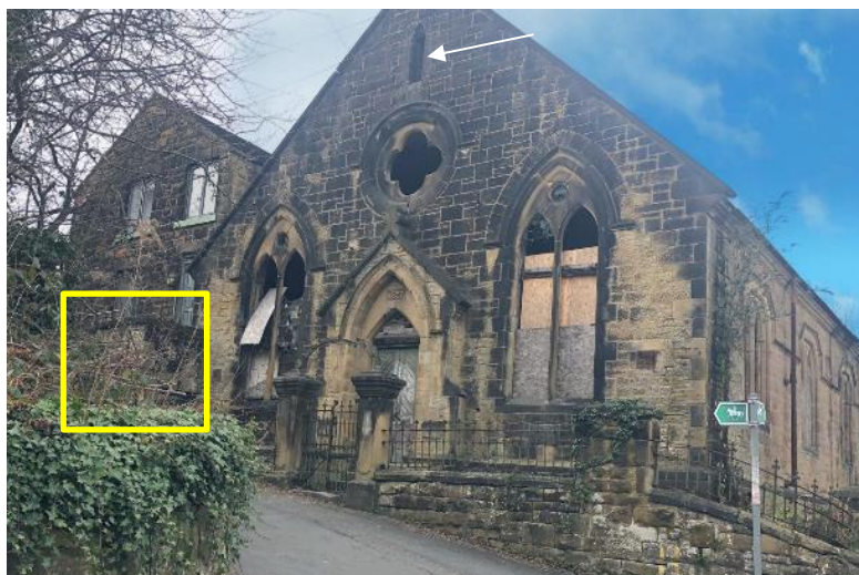
FIGURE 2.3 – SOUTHERN GABLE OF CHAPEL – SHOWING AREA 'A' (YELLOW), 'SLIT' FOR EMERGENCE (WHITE ARROW) AND OPEN CLOVER FEATURE AND WINDOWS
