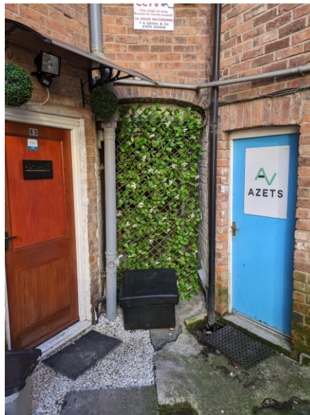
Fig. 6 – Rear door and neighbour's canopy
