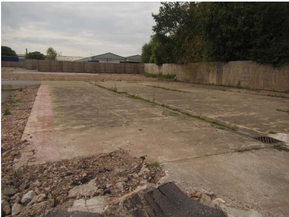
Photograph 24 – Example of hardstanding on site.
