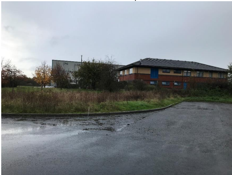
Office block from Ash Road South, along with the unused site entrance
