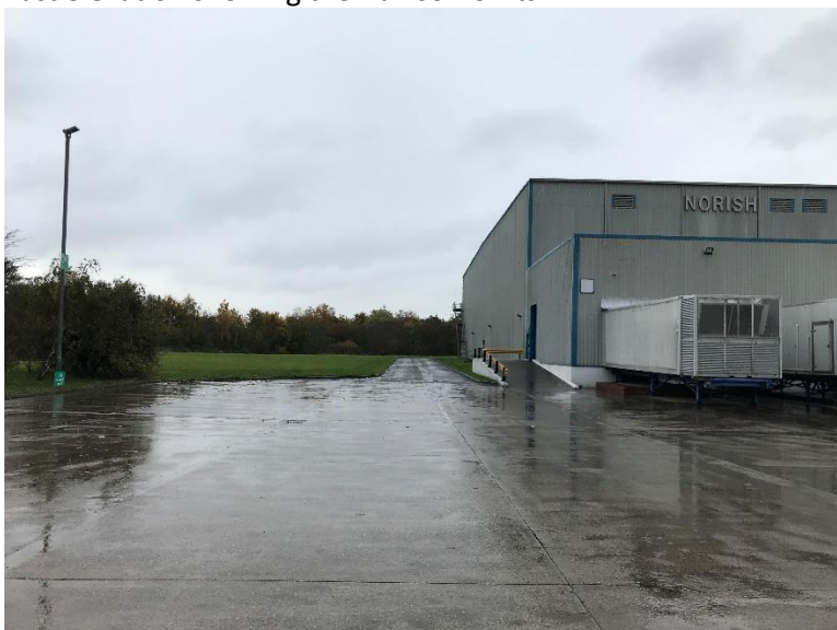
Access road along the western elevation
