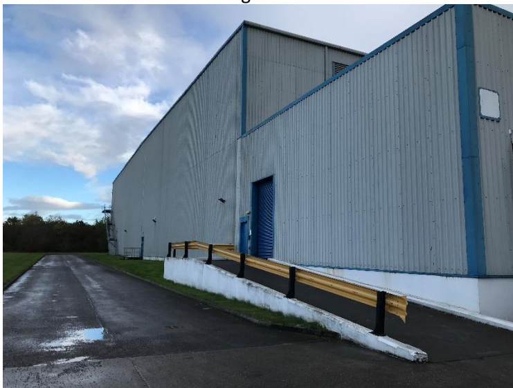
West elevation of the cold store building
