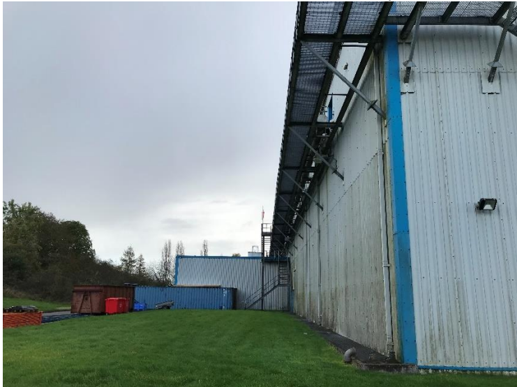
Rear of the cold store building
