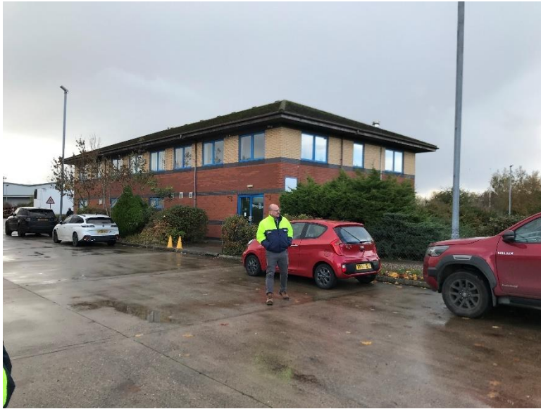
Office block viewed from the service yard
