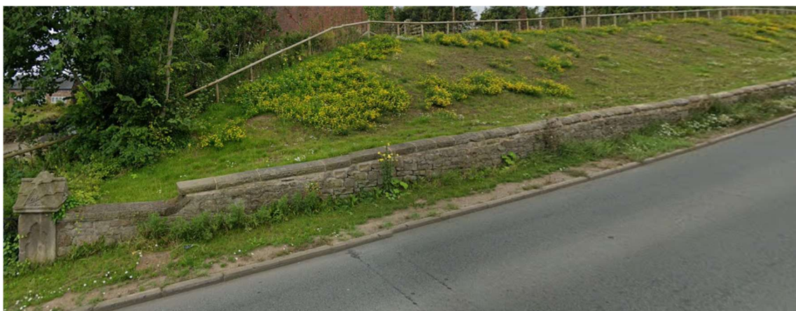
Boundary wall to development site
