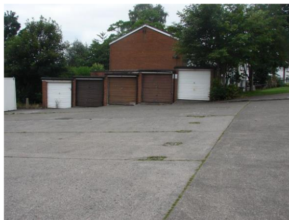
Plate 2: Site B showing hard-standing and garages.
