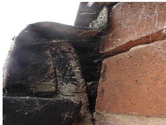
Plate 4: Single gap between wall and timber roof structure of the garages at Site B. Note presence of cobwebs indicating no bat has accessed the garage through this gap.
