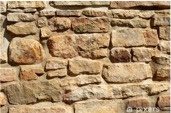
Low level stone wall
