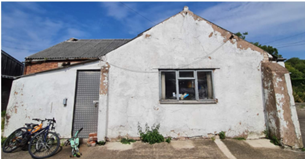
Figure 5: View of Rear Elevation
