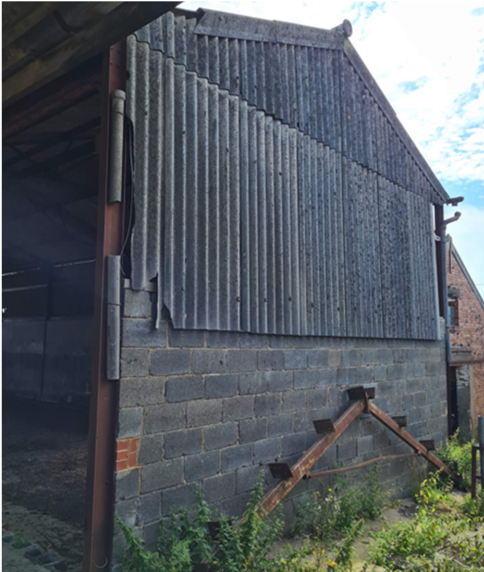
Figure 3: View of Rear Elevation
