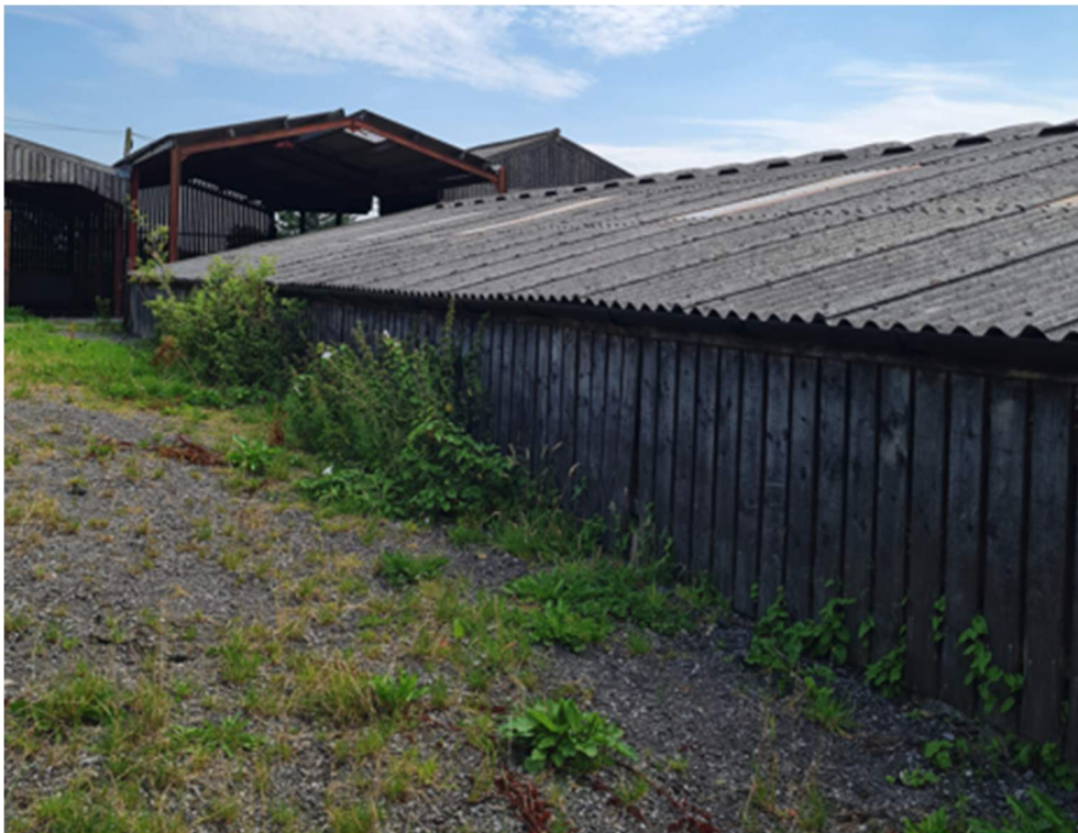
Figure 7: View of Rear Elevation
