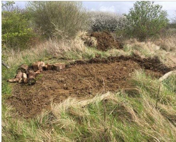
Step 1 – Scraping off topsoil and excavating depression
