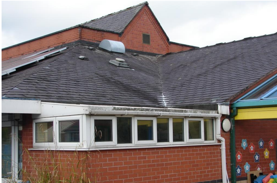
Northeast gable end.
