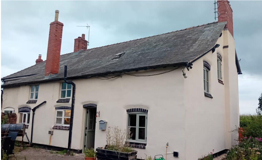
Plate 1: Woodlands Farm showing north (rear) elevation where work is planned
