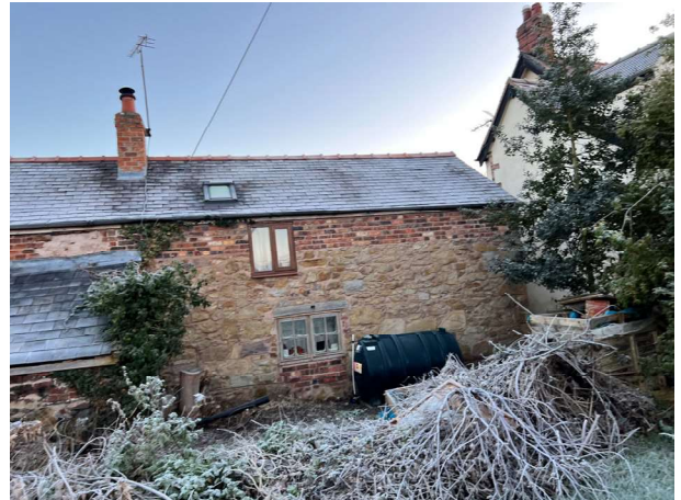
Photograph 7: View to the south east across the current car park
