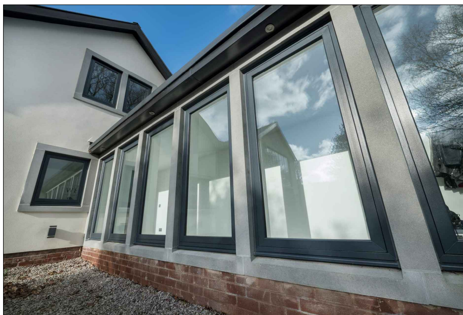
UPVC FLUSH CASEMENT WINDOWS IN GRAPHITE GREY WITH OFF WHITE SMOOTH RENDER.
