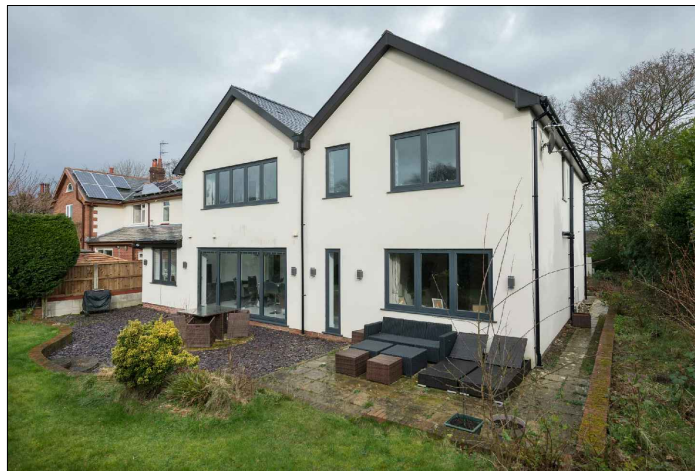
UPVC FLUSH CASEMENT WINDOWS IN GRAPHITE GREY WITH OFF WHITE SMOOTH RENDER.
