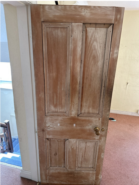
IN-DR-032 - Door removed and stored securely
