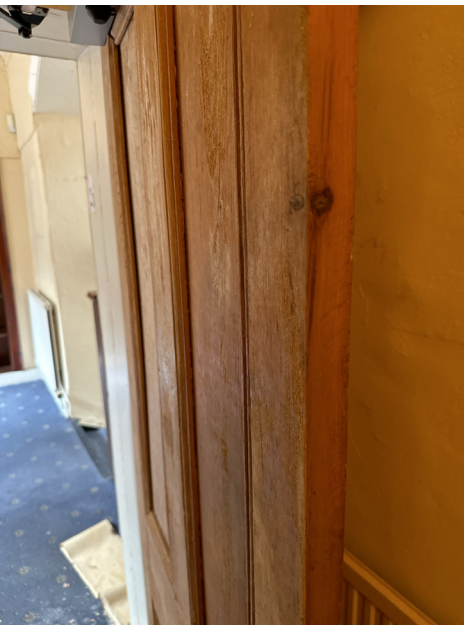
IN-DR-016 - Door retained and blocked up to reveal side as per Retained Existing door detail drawing 1268-03-32-004
