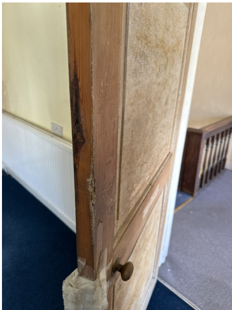
IN-DR-028 - Door retained and blocked up to reveal side as per Retained Existing door detail drawing 1268-03-32-004
