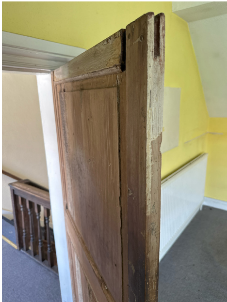
IN-DR-031 - Door retained and blocked up to reveal side as per Retained Existing door detail drawing 1268-03-32-004
