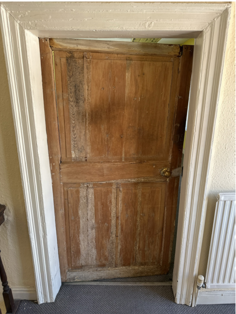
IN-DR-031 - Door retained and blocked up to reveal side as per Retained Existing door detail drawing 1268-03-32-004
