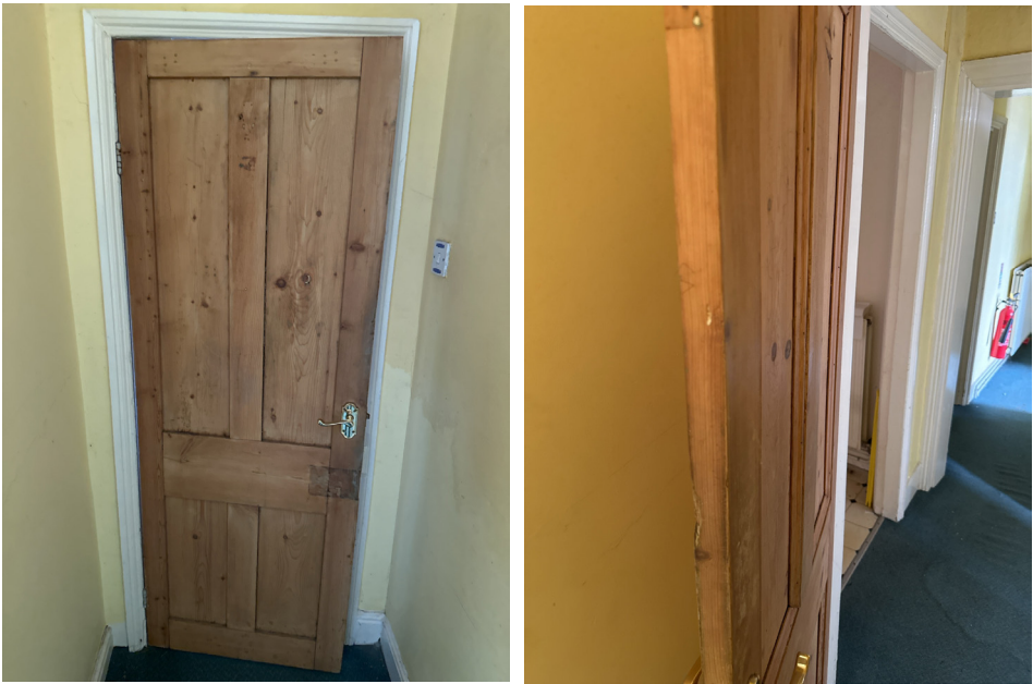
IN-DR-026 - Door removed and stored securely
