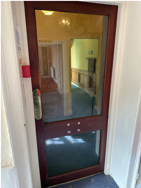
IN-DR-024 - Door removed and disposed of
