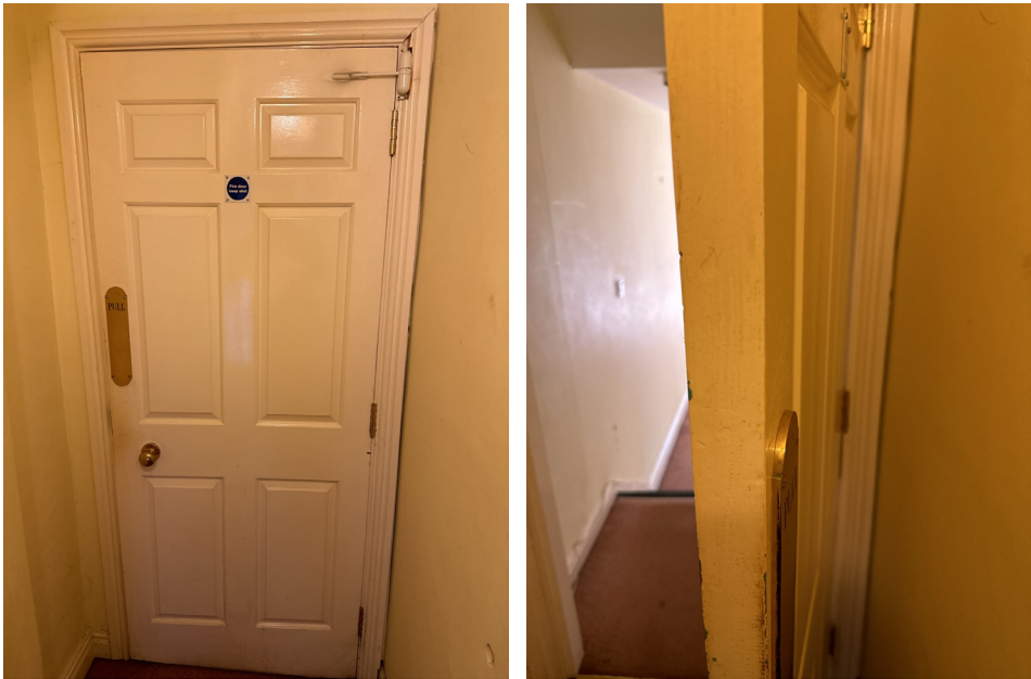
IN-DR-021 - Door removed and disposed of. Door to modern partition wall
