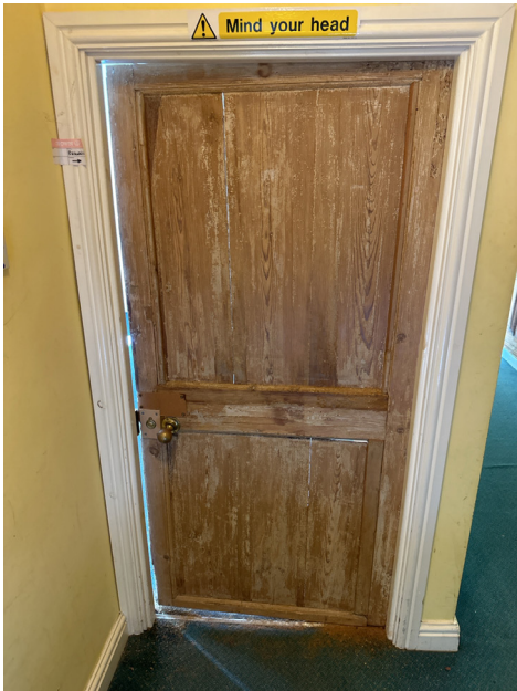
IN-DR-025 - Door removed and stored securely
