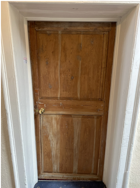
IN-DR-018 - Door retained and blocked up to reveal side as per Retained Existing door detail drawing 1268-03-32-004
