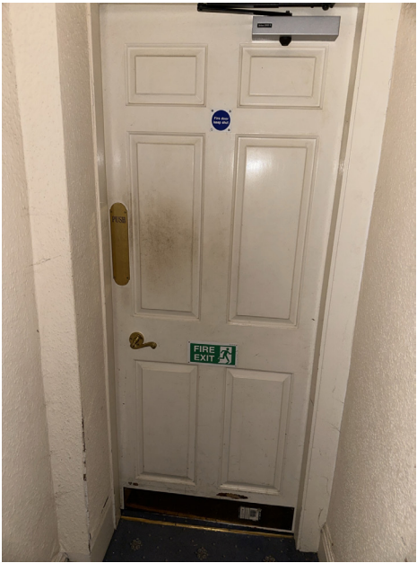
IN-DR-004 - Door removed and disposed of
