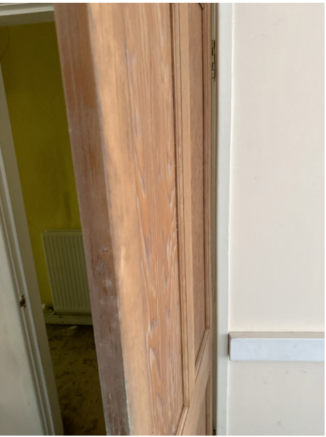
IN-DR-011 - Door retained and blocked up to reveal side as per Retained Existing door detail drawing 1268-03-32-004
