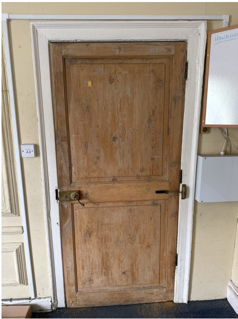
IN-DR-005 - Door Removed and stored securely
