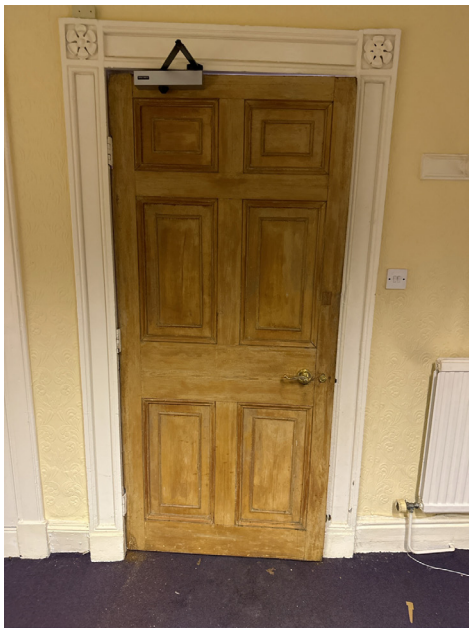
IN-DR-008 - Door removed and stored securely
