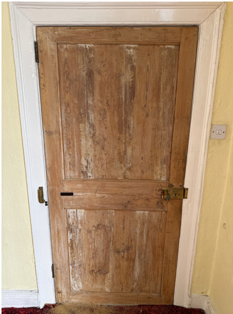
IN-DR-016 - Door retained and blocked up to reveal side as per Retained Existing door detail drawing 1268-03-32-004
