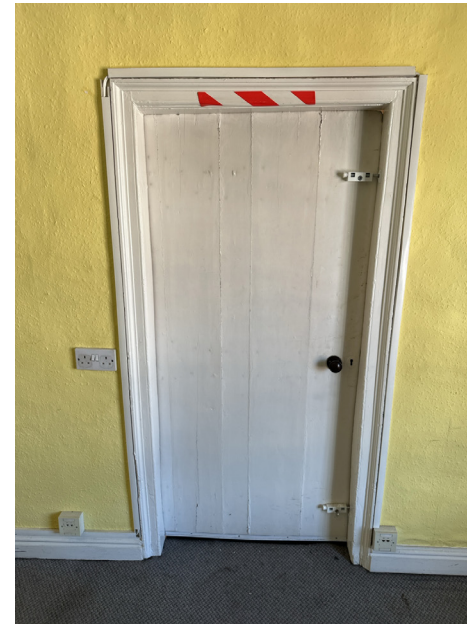
IN-DR-033 - Door removed and stored securely
