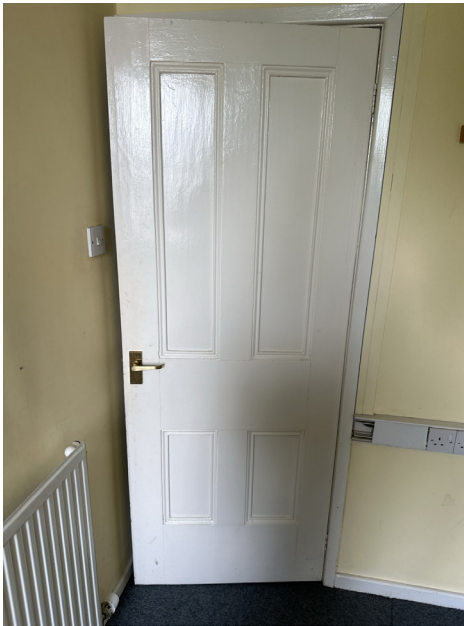
IN-DR-015 - Door removed and disposed of
