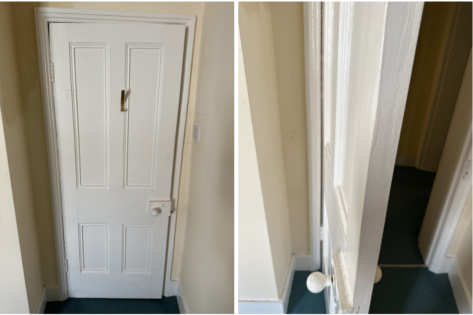
IN-DR-027 - Door removed and stored securely
