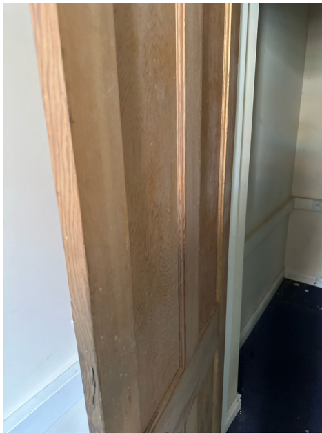
IN-DR-009 - Door retained and blocked up to reveal side as per Retained Existing door detail drawing 1268-03-32-004
