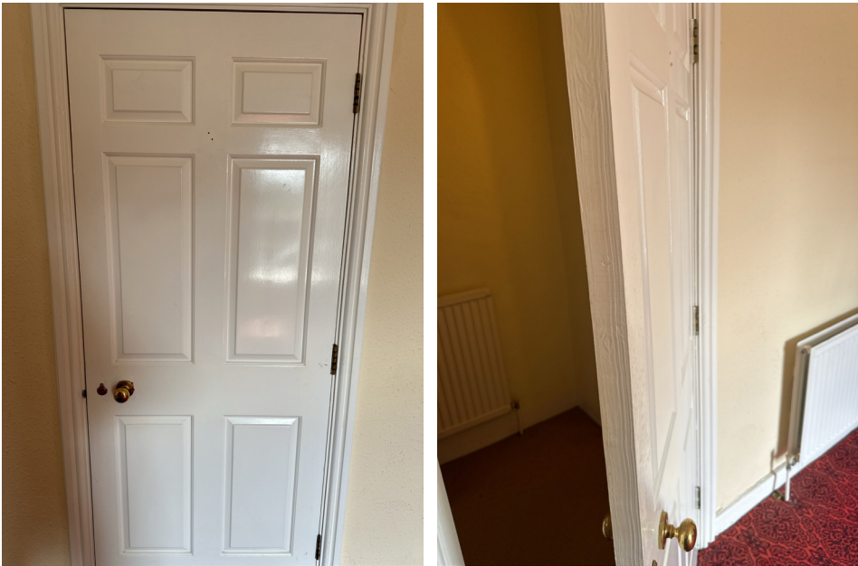
IN-DR-020 - Door removed and disposed of. Door to modern partition wall
