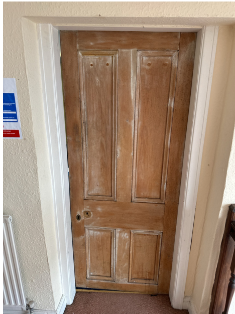
IN-DR-030 - Door removed and stored securely
