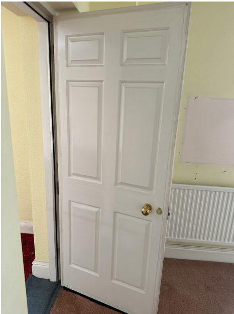
IN-DR-017 - Door removed and stored securely
