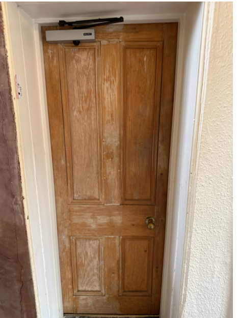
IN-DR-019 - - Door removed and stored securely
