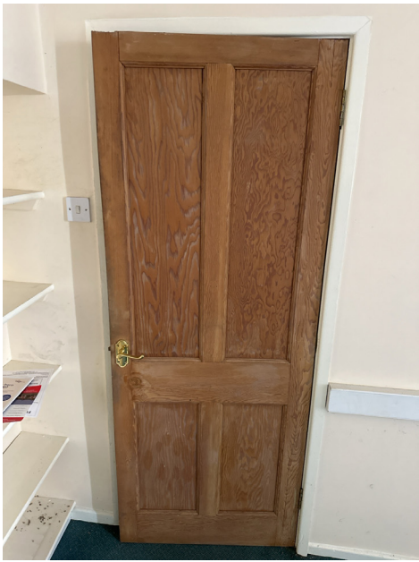
IN-DR-011 - Door retained and blocked up to reveal side as per Retained Existing door detail drawing 1268-03-32-004
