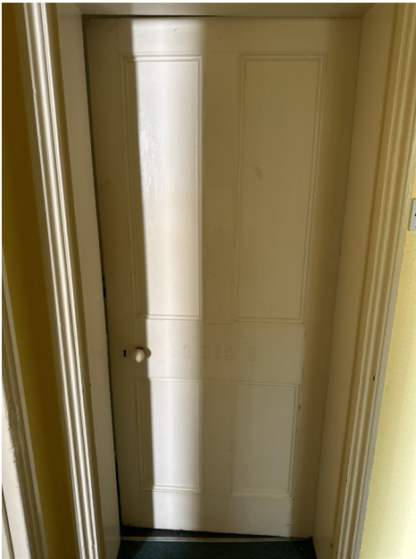
IN-DR-014 - Door removed and stored securely
