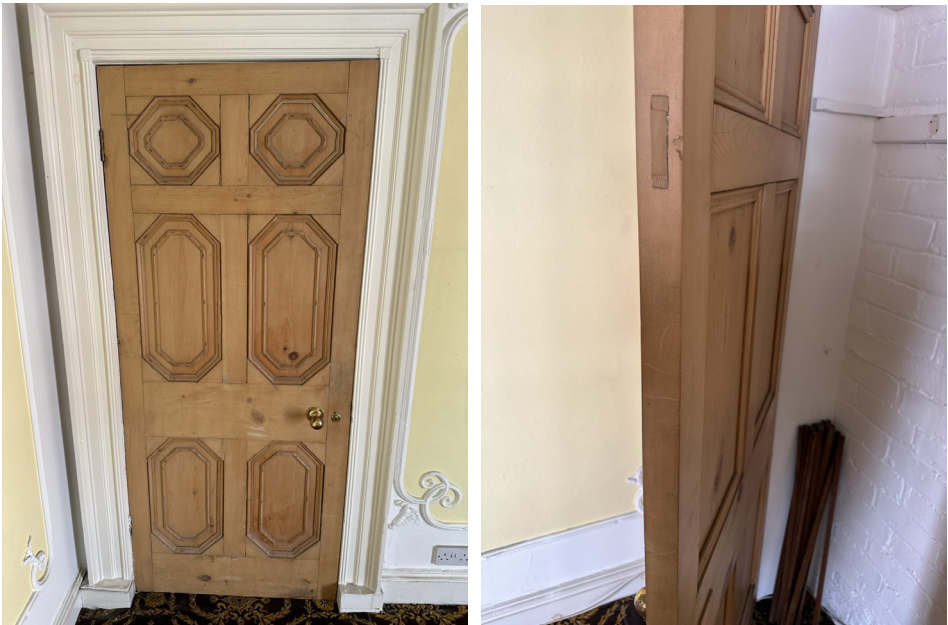
IN-DR-023 - Door removed and stored securely
