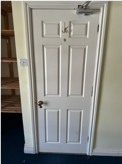
IN-DR-029 - - Door removed and disposed of
