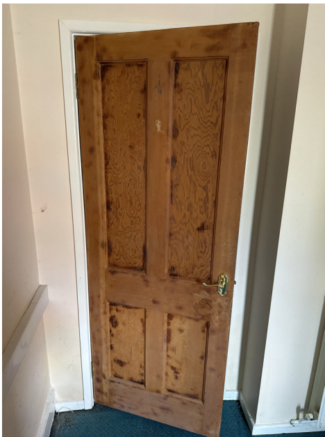
IN-DR-009 - Door retained and blocked up to reveal side as per Retained Existing door detail drawing 1268-03-32-004
