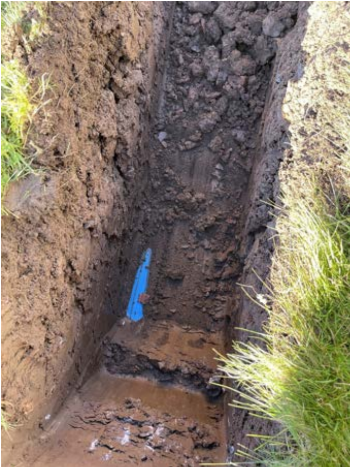
TP103 utility and pit
