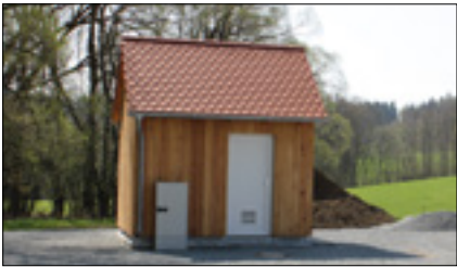
Example: Installation in a machine house
