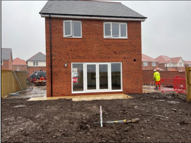
Photographs 1 & 2: Showing the depth of the inert cover and location of the validation hole within the rear garden of Plot 348 and the depth of inert cover achieved. Photographs taken 3 rd March 2022.
