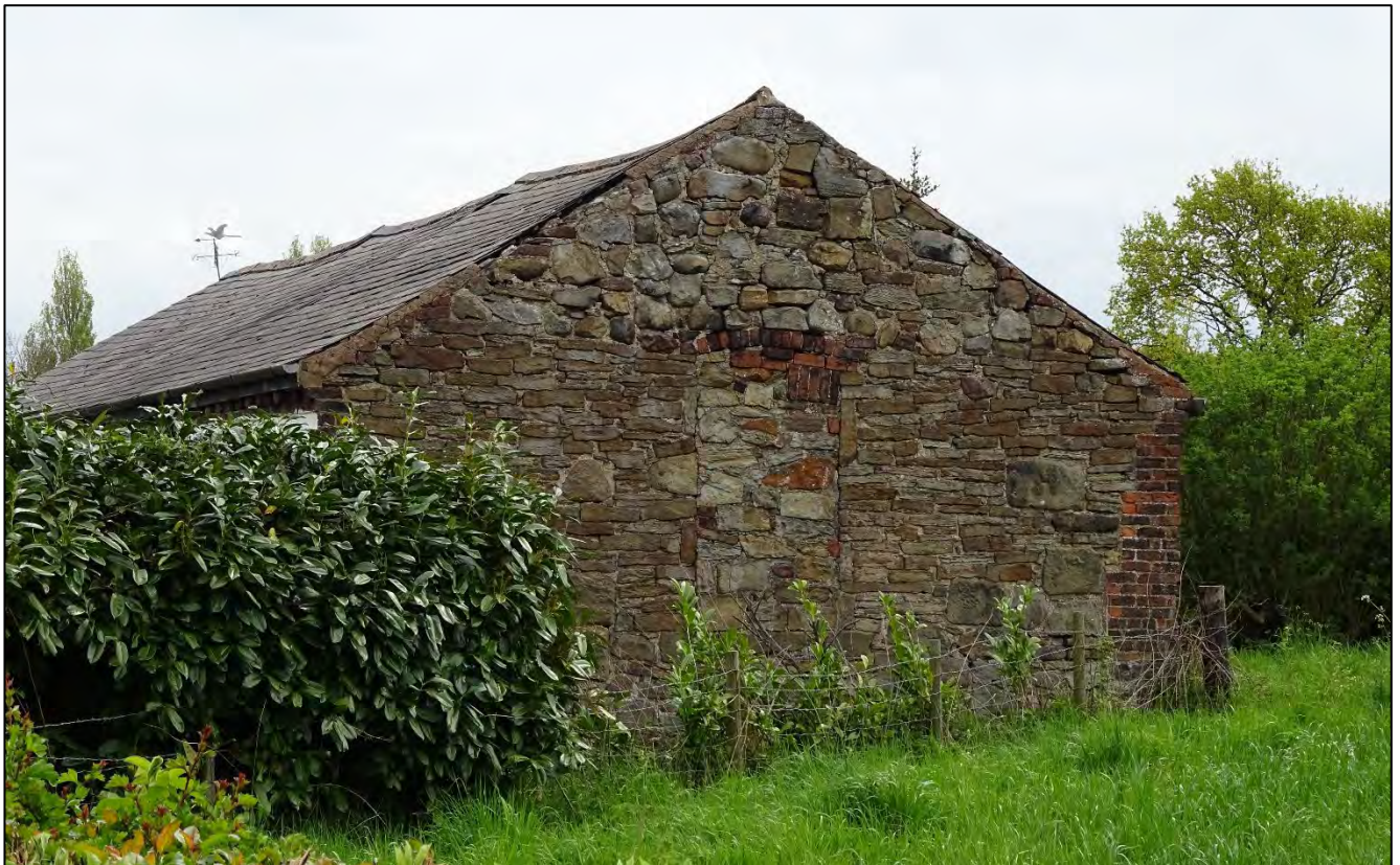
Plate 15. West-facing elevation of barn, looking south-east.
