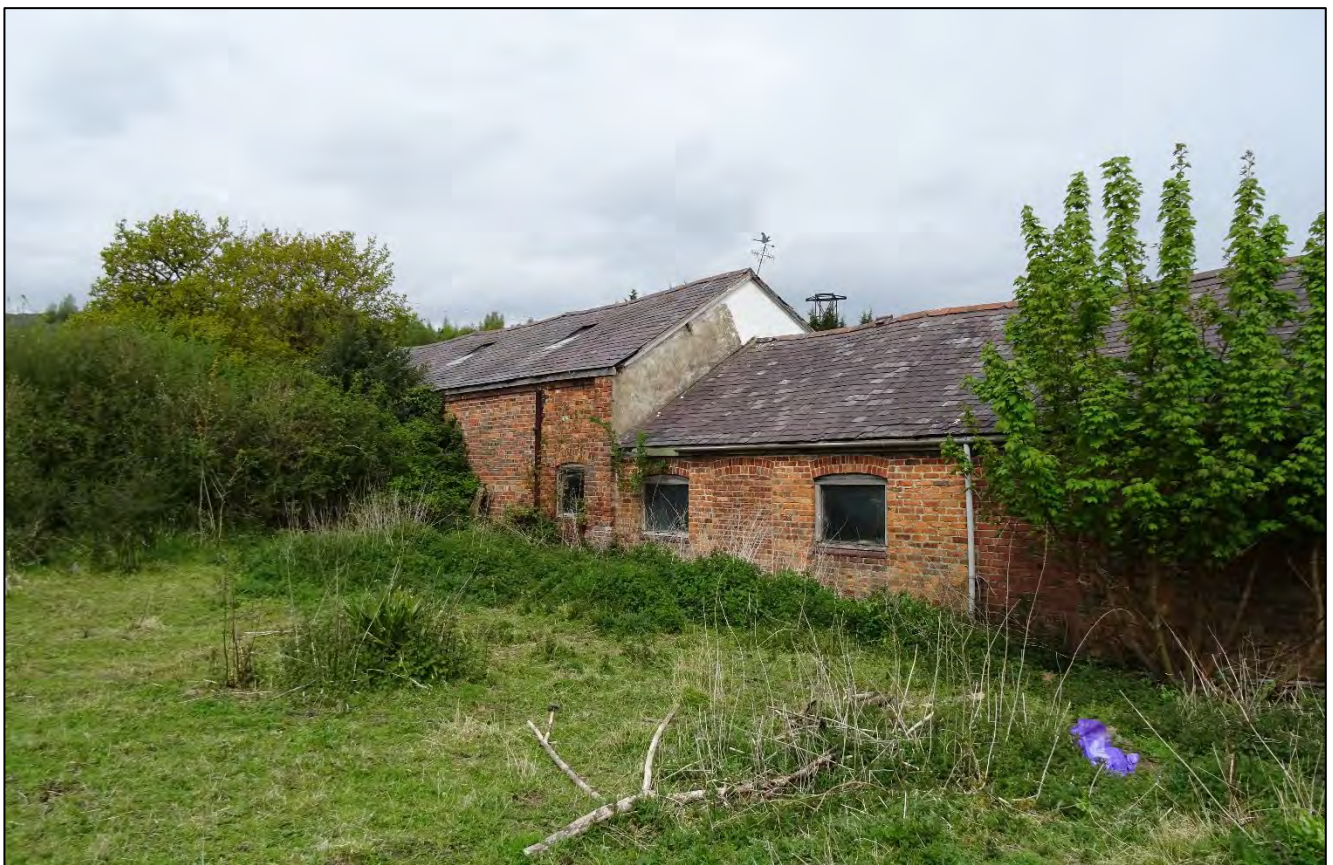
Plate 13. East- and south-facing elevations of barn with single storey adjoining barn to the east, looking north-west.
