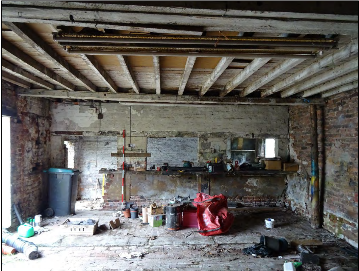
Plate 16. Interior of barn, looking east to later dividing wall. 2m scale.
