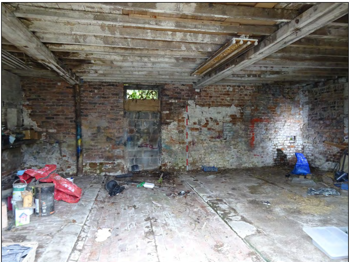
Plate 17. Rear wall of barn, looking south. 2m scale.
