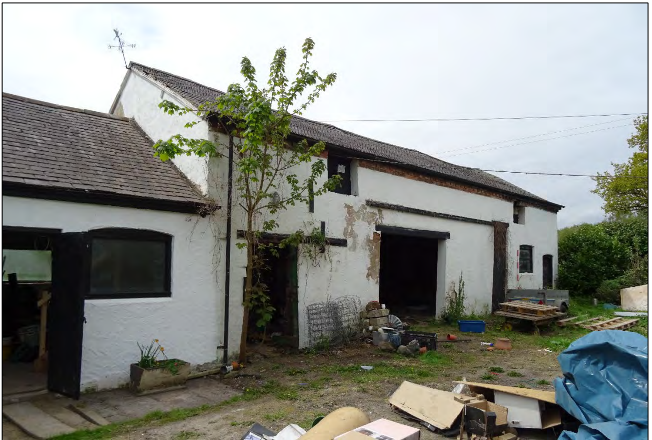
Plate 2. Front elevation of barn, looking south-west.
