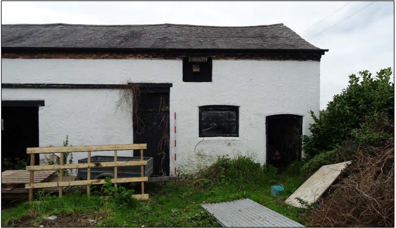
Plate 3. West end of front elevation of barn, looking south. 2m scale.
