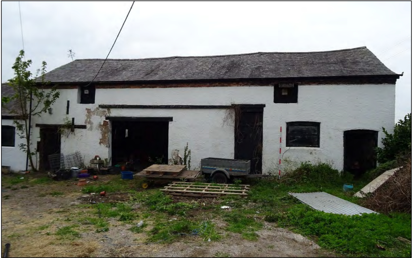
Plate 1. Front (north-facing) elevation of Plas Grono Farm barn, looking south. 2m scale.
