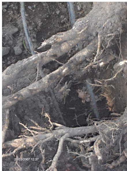
Typical root damage caused by excavation works
