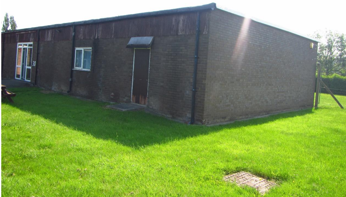
Photograph 2 – Southern aspect of Building 1.
