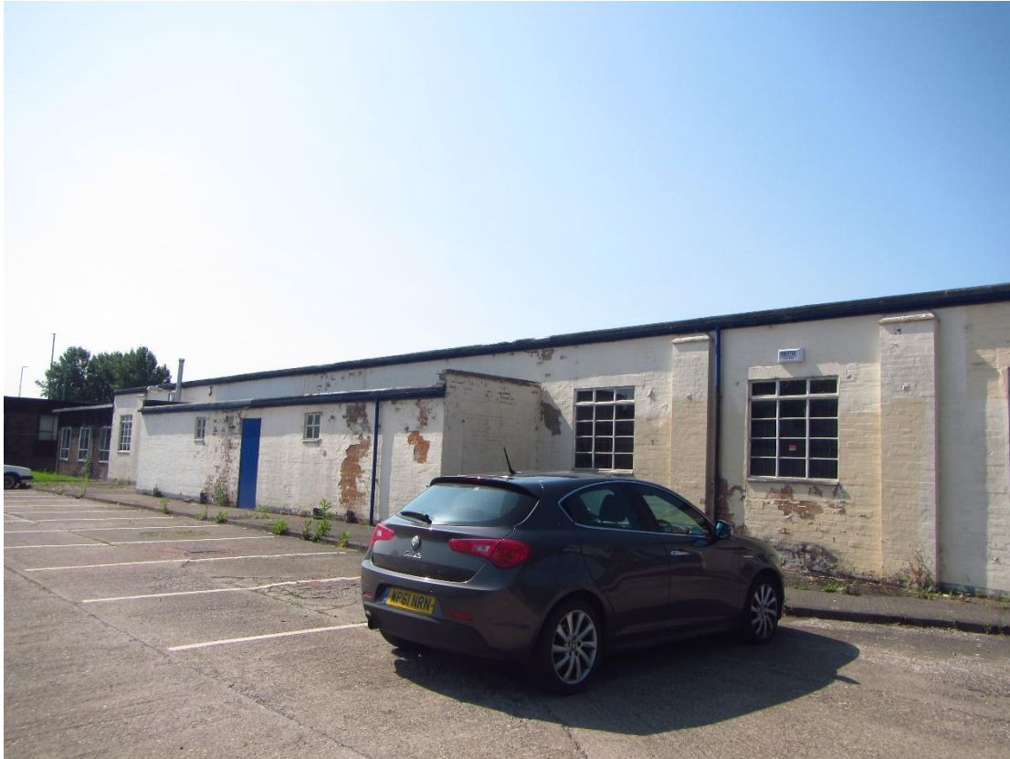
Photograph 5 – Northern aspect of Building 2.
