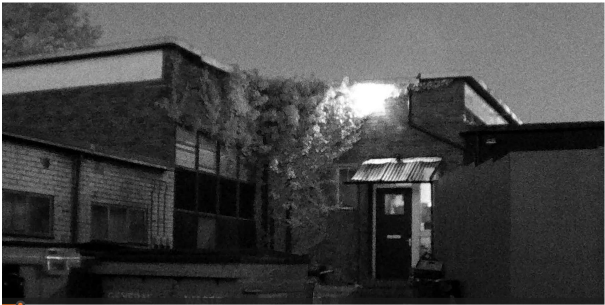
Camera Viewpoint 4 – Southwestern aspect of Building 1 on 17/06/2024.
