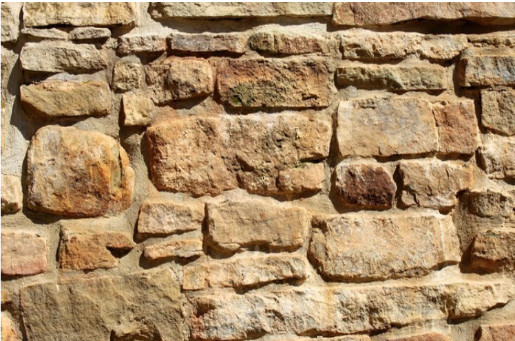
Low level stone wall
