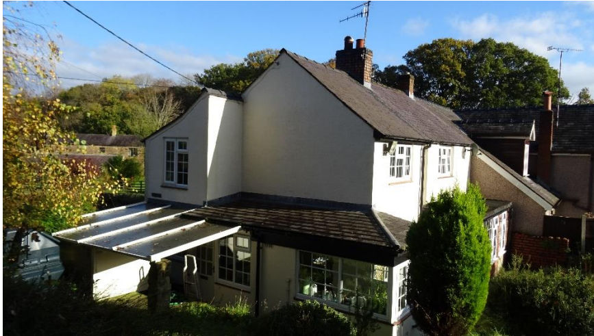
Figure 4.2. House from southwest
