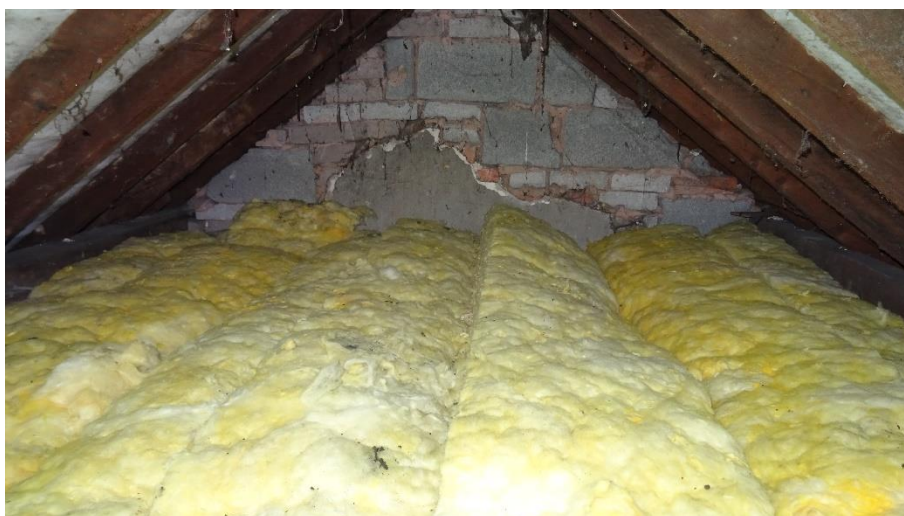
Figure 4.8. Clean insulation in eastern loft
