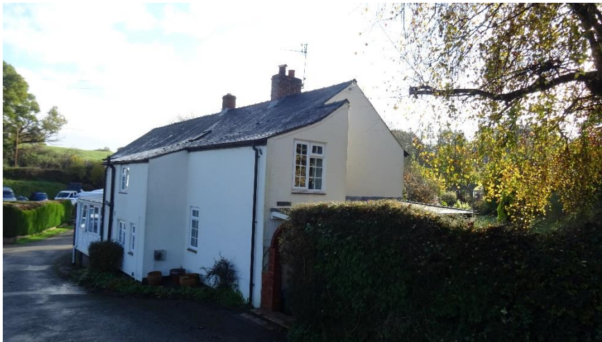
Figure 4.3. House from northwest
