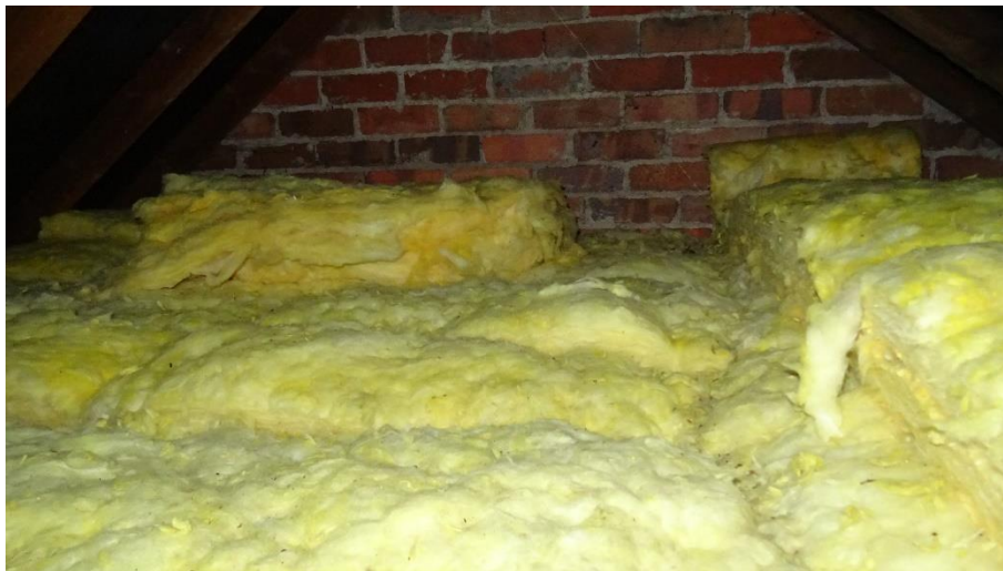
Figure 4.7. Clean insulation in western loft
