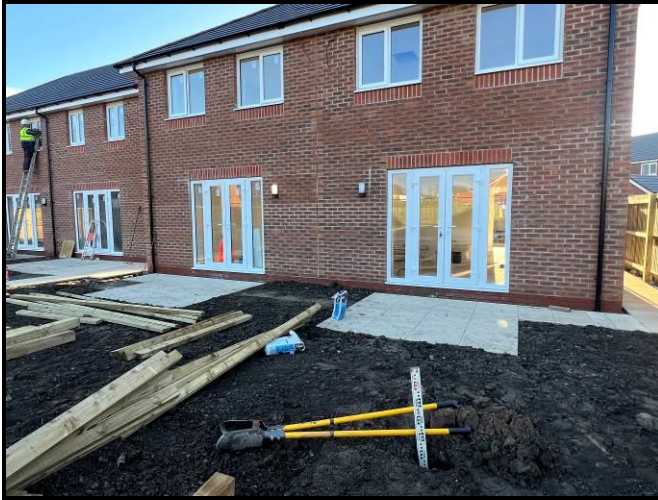
Photographs 1 & 2: Showing the location of the validation hole within the rear garden of Plot 246 and the depth of inert cover achieved. Photographs taken 23 rd November 2023.
