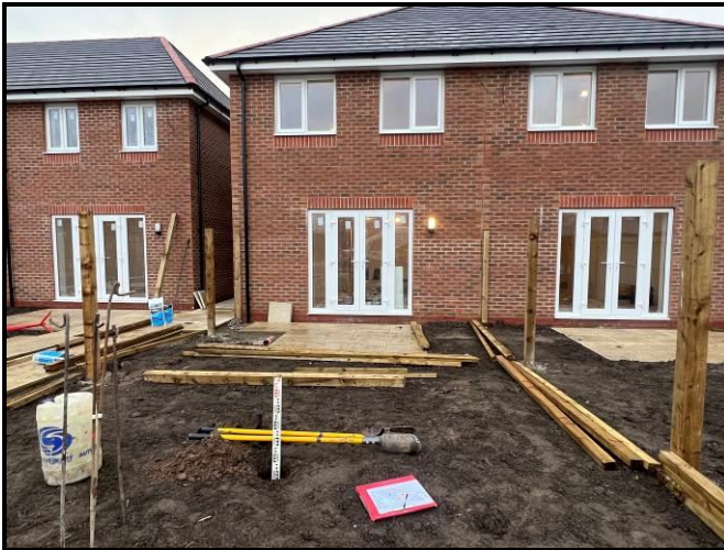
Photographs 4 & 5: Showing the location of the validation hole within the rear garden of Plot 247 and the depth of inert cover achieved. Photographs taken 24 th November 2023.
