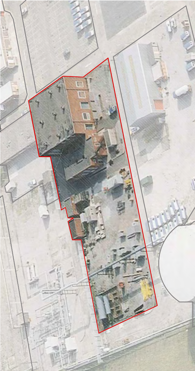
Training Centre of WWU - highlighted aerial image
