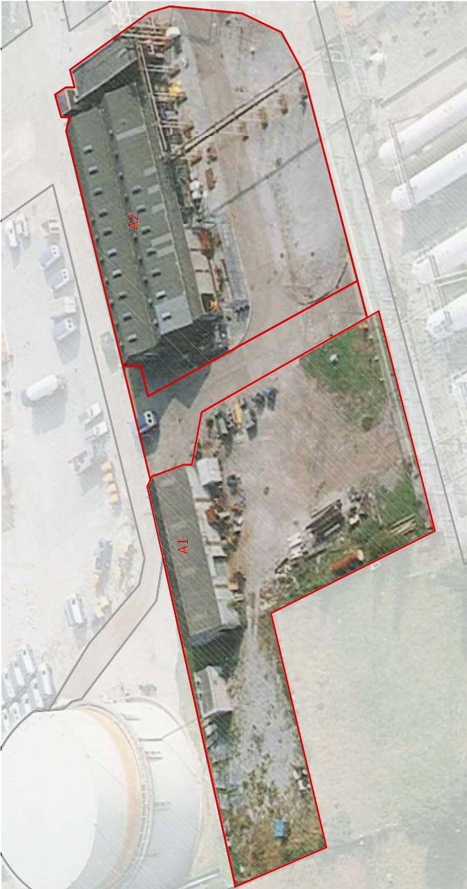
Welding workshop & Store - highlighted aerial image
