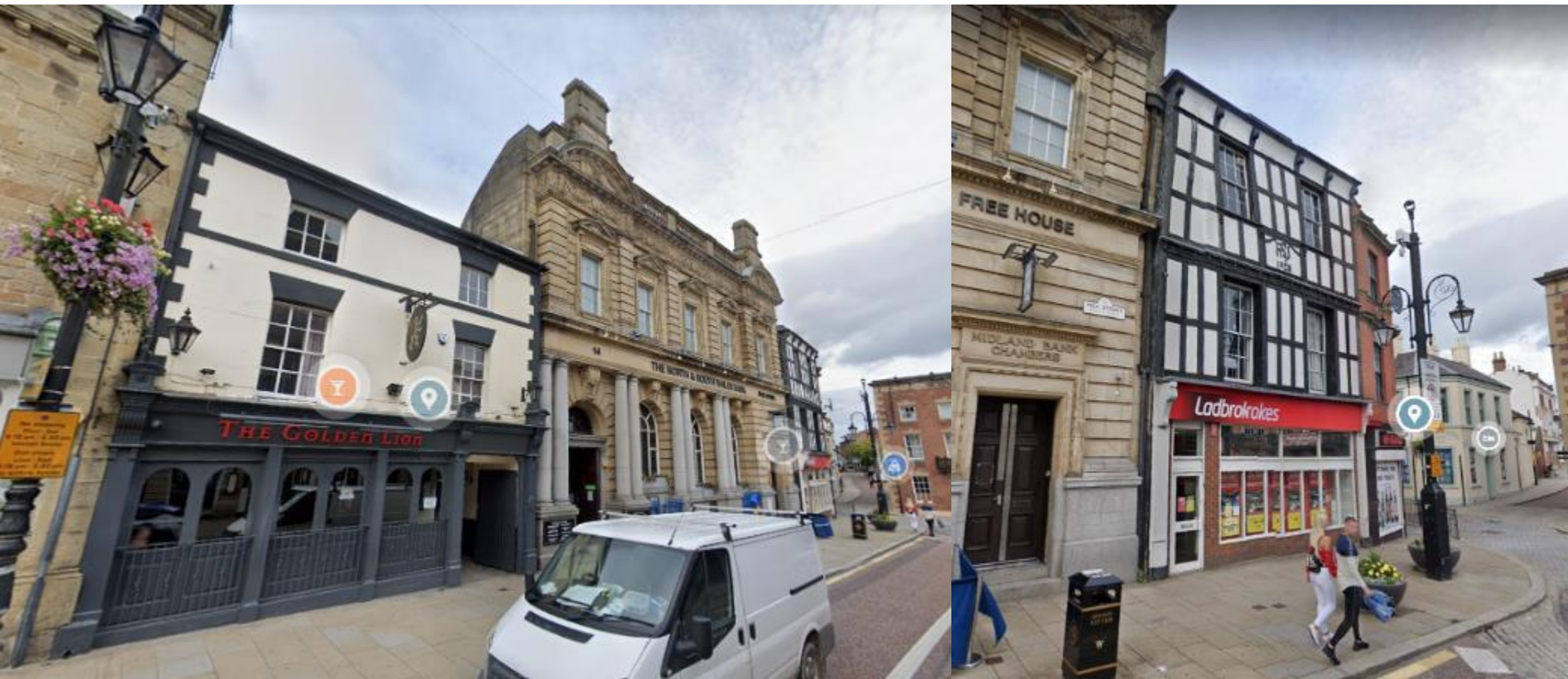
View of 14 High Street with the neighbouring buildings either side.
