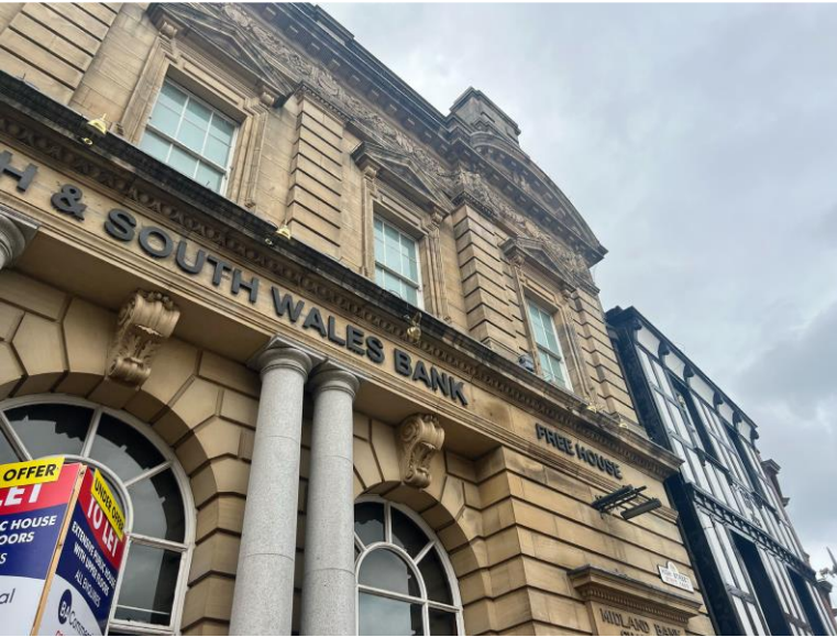
Images of existing windows
