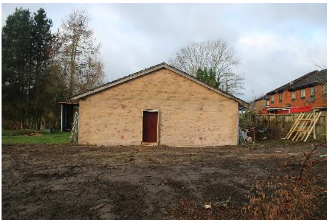
Photo 4— Eastern Gable of Scout Headquarters with scrub, debris and old shipping containers removed
