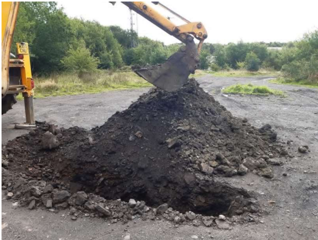
Trial pit 1 - Spoil
