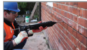
5. Insert a further bead of HeliBond over the exposed HeliBar, finishing 2mm from the face, and 'iron' firmly into the slot using the HeliBar Insertion Tool
