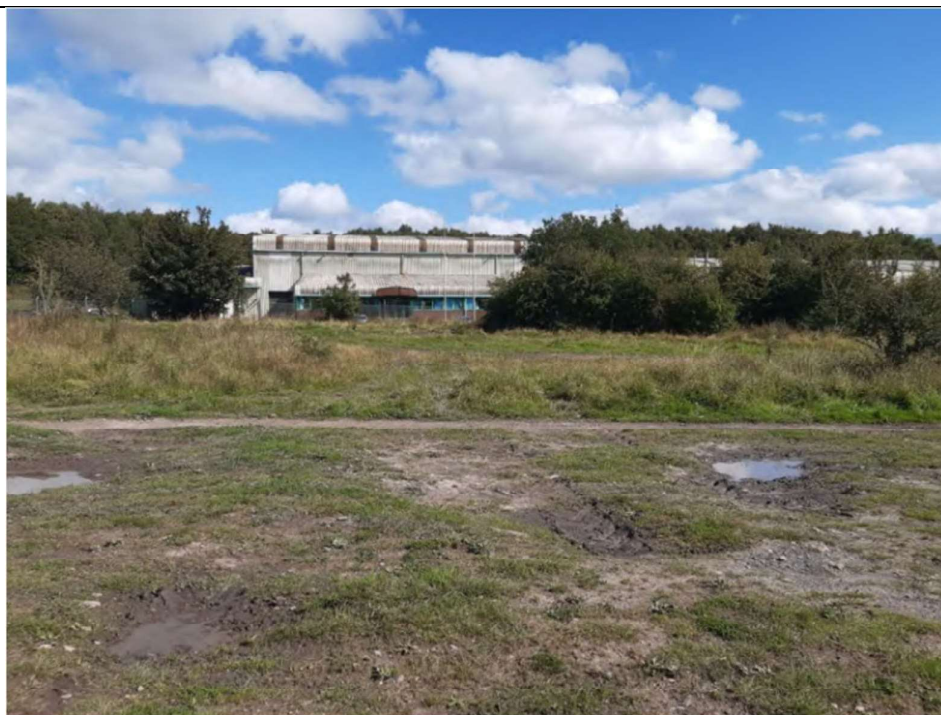
Photo 3 - Northern side of the site facing east
