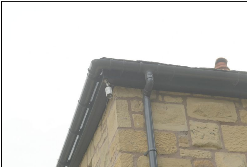
Soffits at the side and front are sealed
