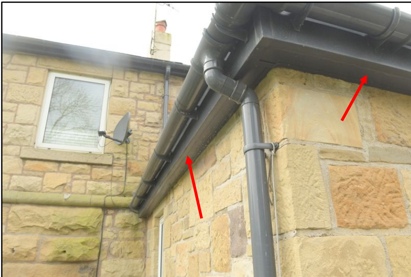
Intact and sealed soffits
