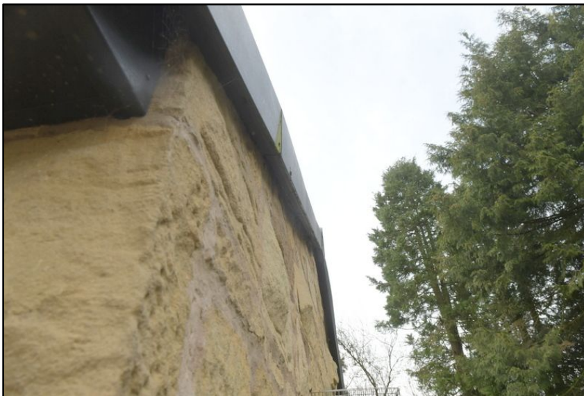
Gable fascia is sealed with no gaps
