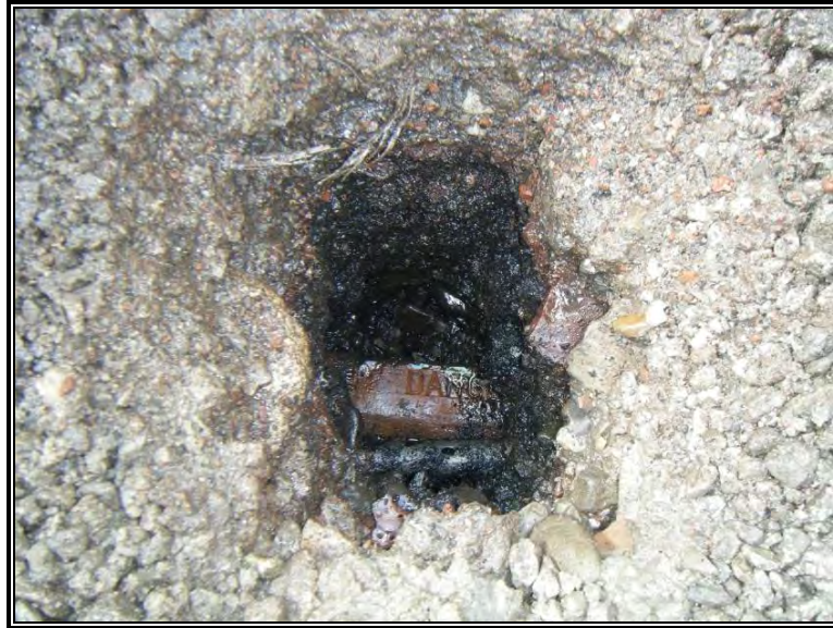
Plate 7. Contamination encountered during service location using vacuum excavation.
