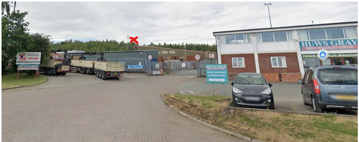
Figure 2: View of the site from the road frontage.
