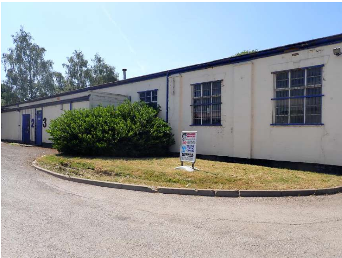
Photograph 18 – Northeastern aspect of Building 4.
