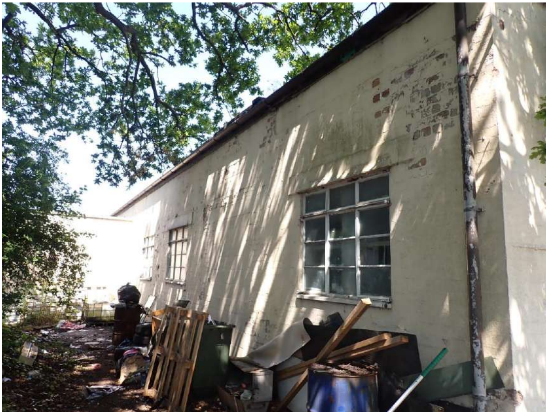
Photograph 20 – Southwestern aspect of Building 4.
