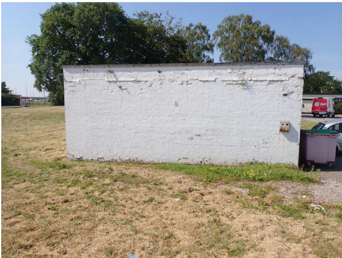
Photograph 6 – Northeastern aspect of Building 2.
