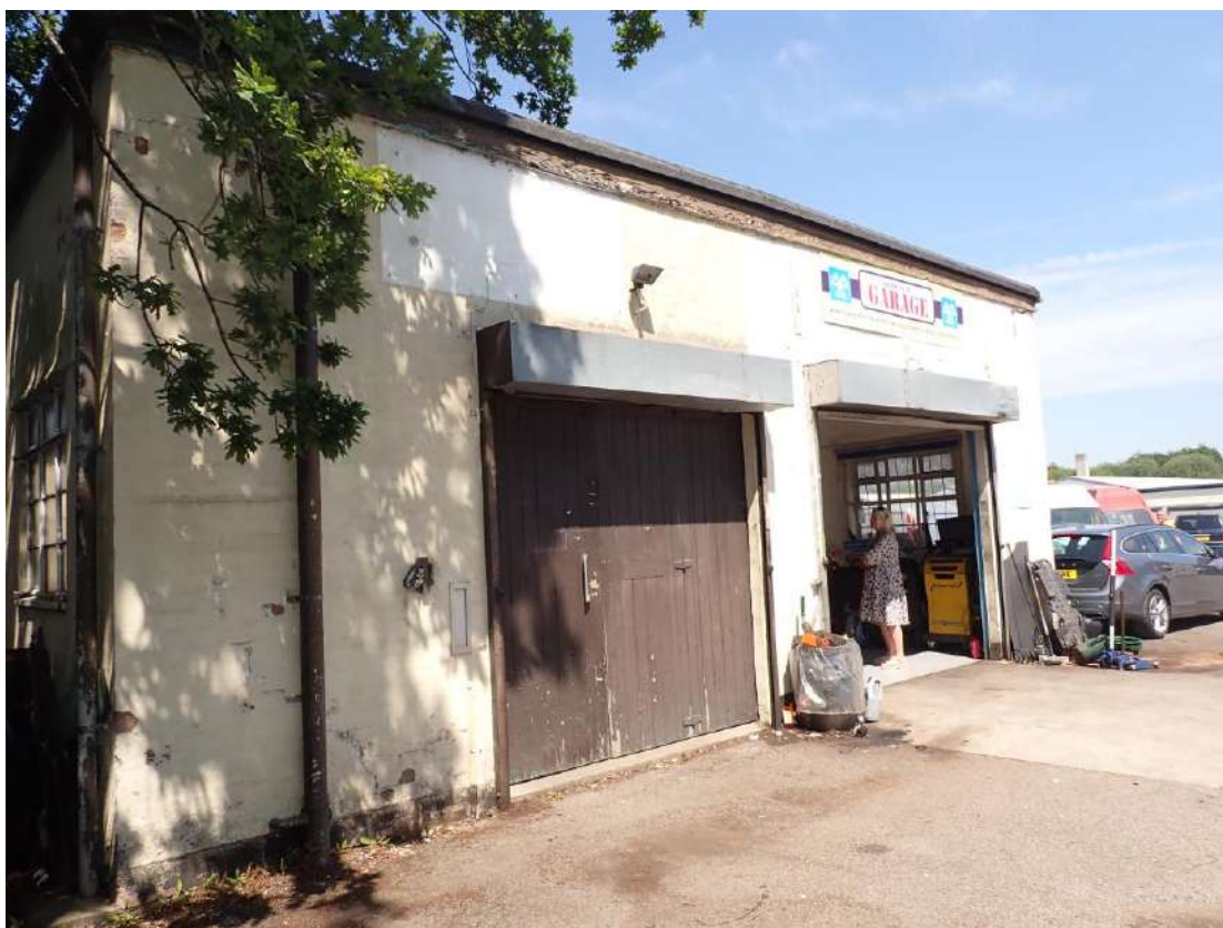
Photograph 21 – Southeastern aspect of Building 5.
