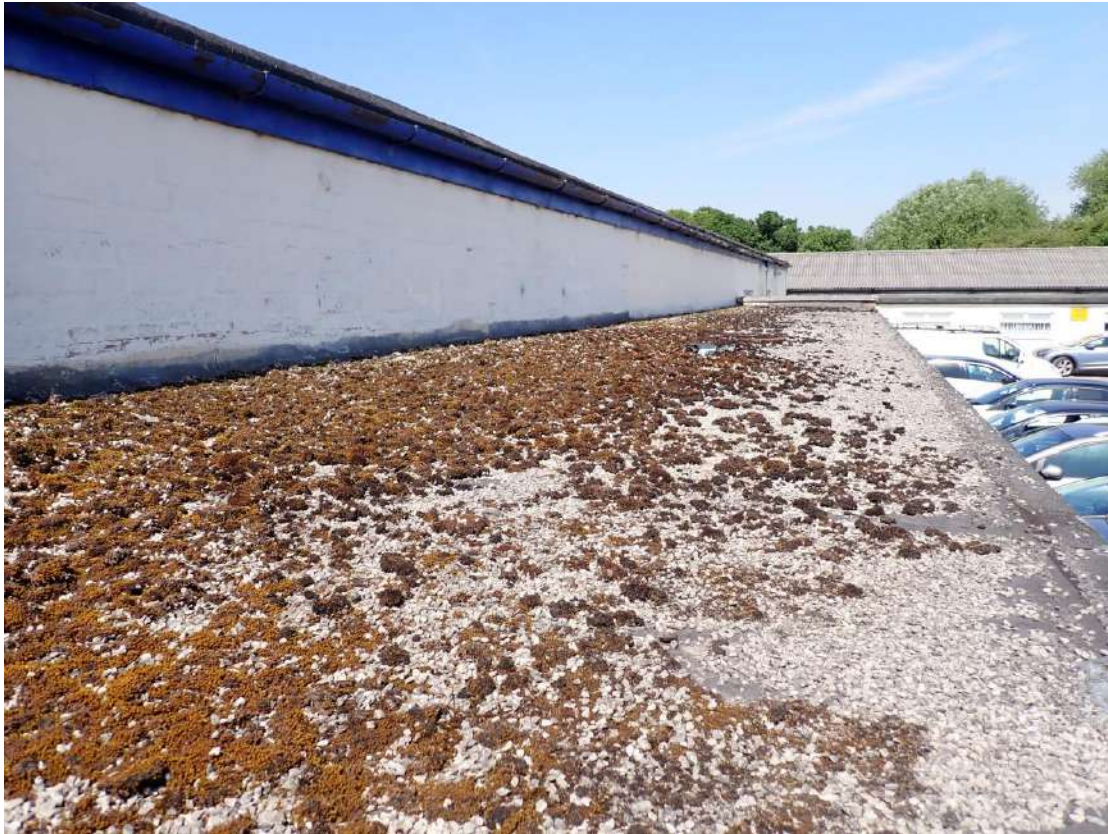
Photograph 13 – Northeastern aspect of Building 3.
