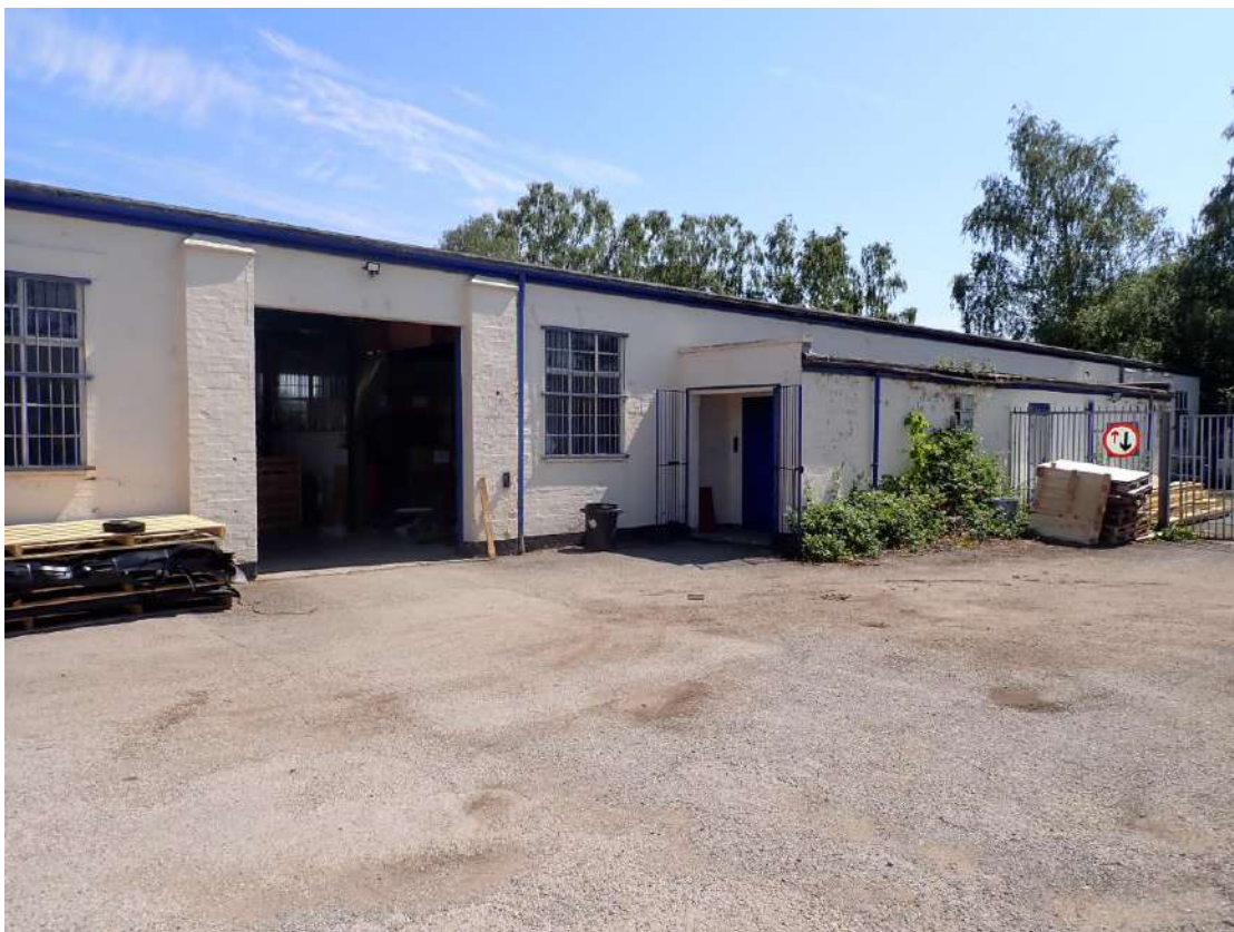
Photograph 14 – Southwestern aspect of Building 4.
