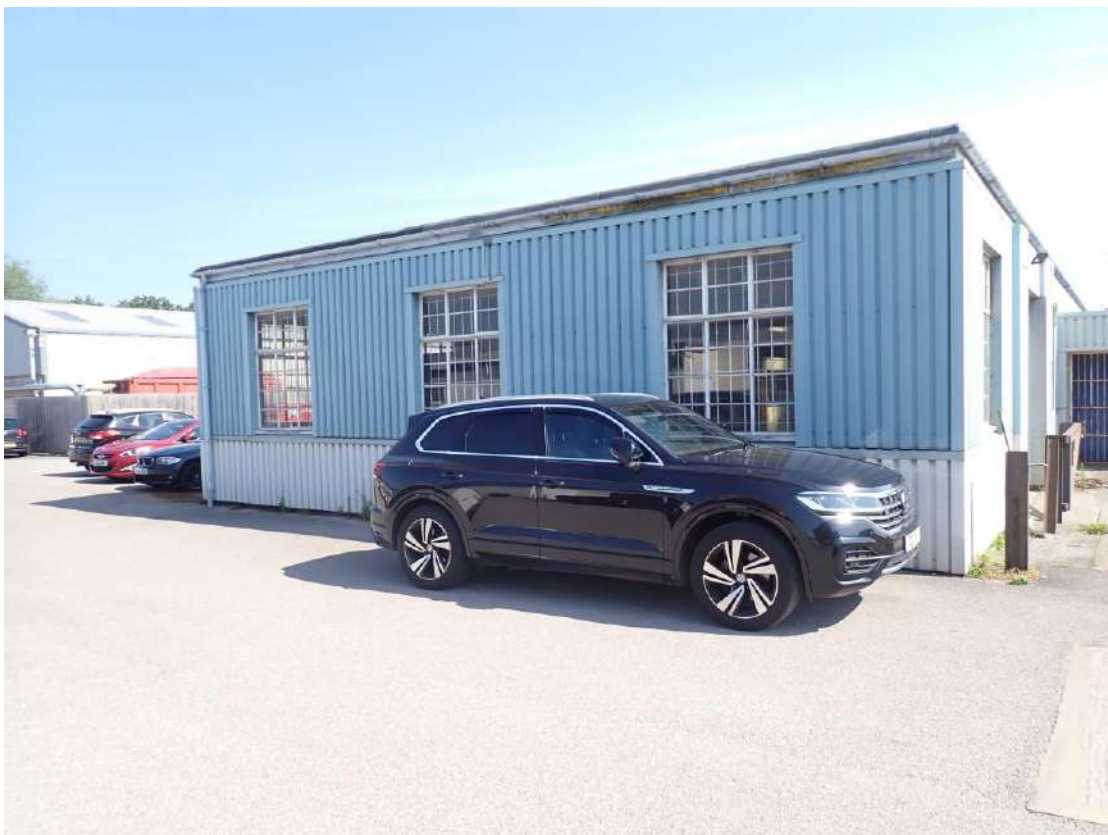
Photograph 2 – Southwestern aspect of Building 1.
