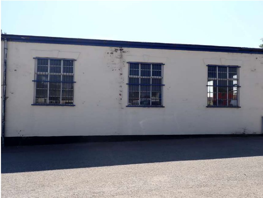
Photograph 17 – Northwestern aspect of Building 4.
